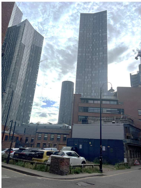
Figure 2 – Photograph of the site with view from corner of Little Peter Street and Constance Street
