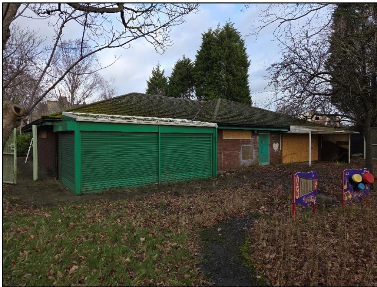
Photograph 1. Showing the southeast elevation
