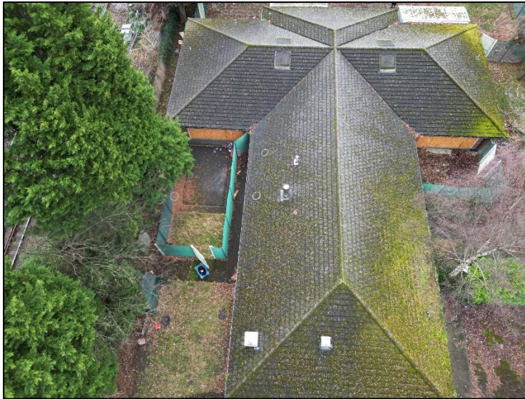
Photograph 2. Showing the roof
