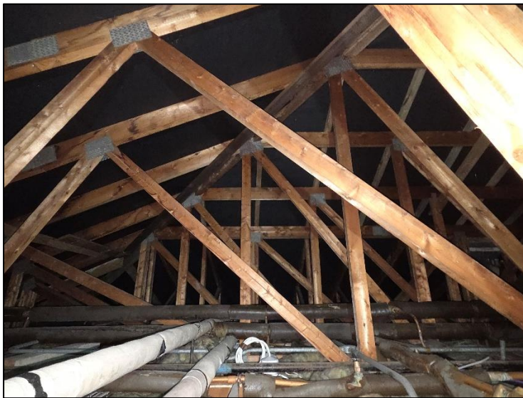
Photograph 5. Showing the roof void.
