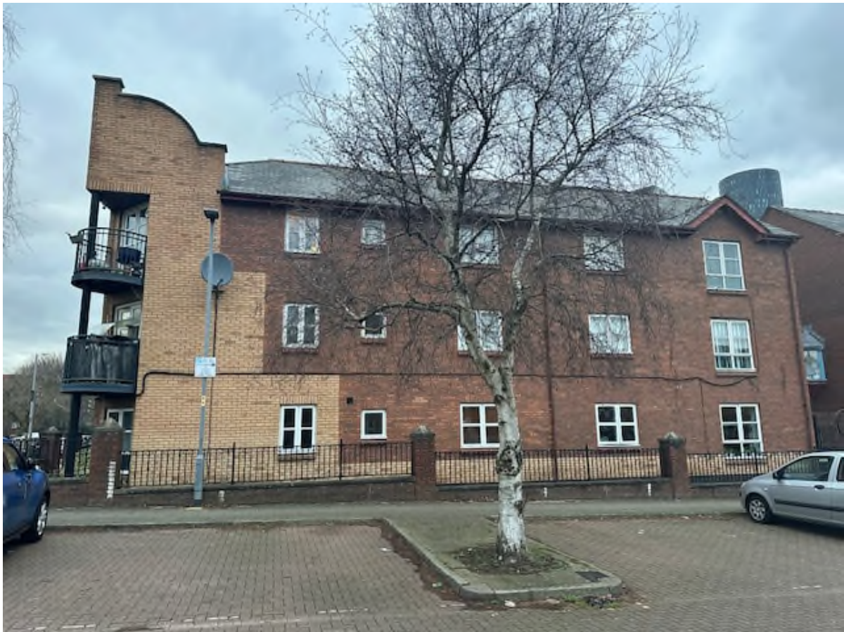
South elevation of the application property fronting Eliza Street
