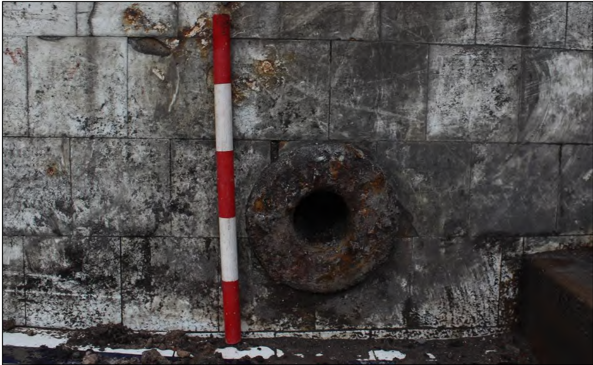
Plate 64: Cast iron collared pipe in pool 225 (0.50m scale)
