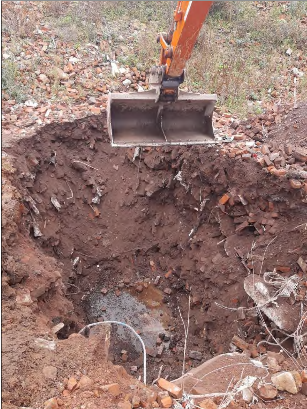
Plate 33: A mid-excavation shot of Trench 9, illustrating that the entirety of the trench had been heavily remediated. Looking south.
