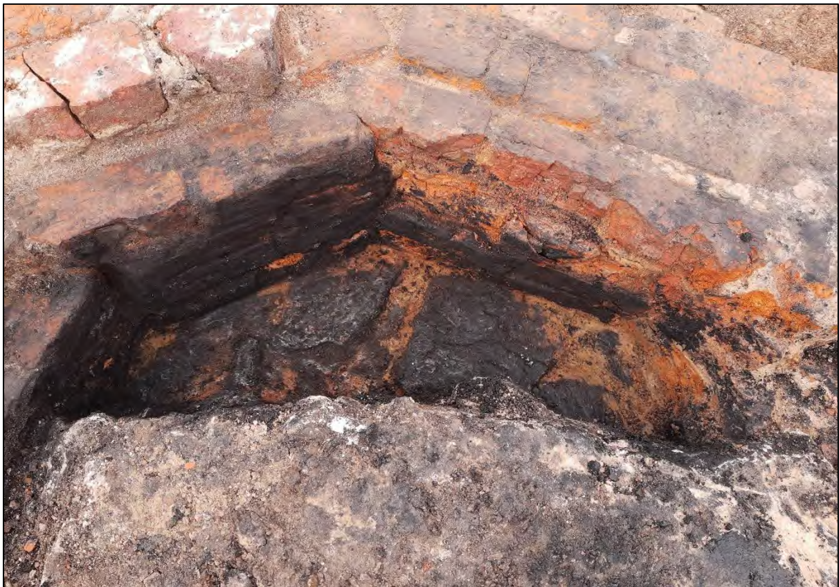
Plate 178: Close-up showing the scorched bedrock base of the chimney 110
