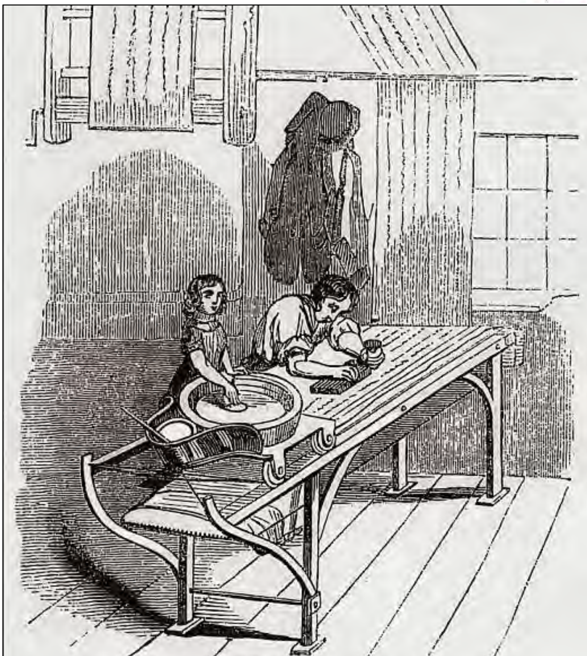
Plate 193: Block-printing a design onto a length of calico cloth
