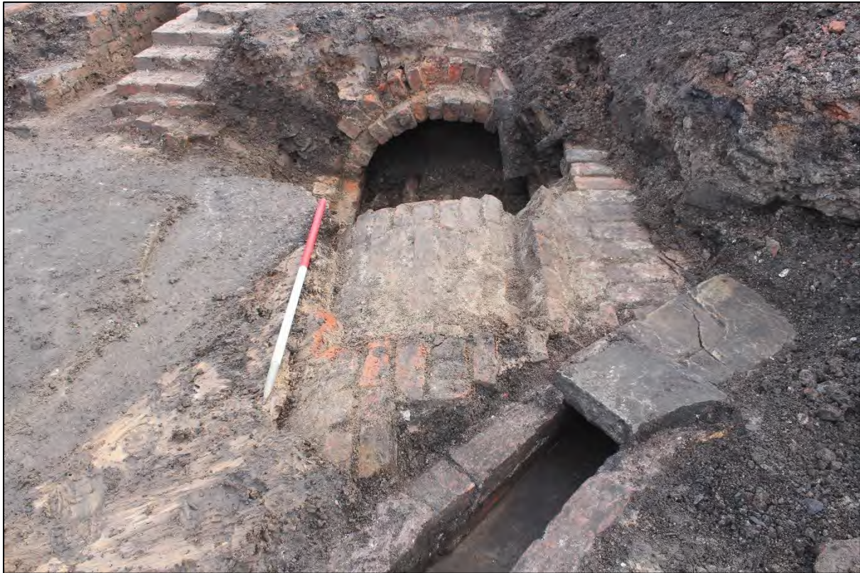
Plate 85: Vaulted culvert 3079 truncated by drain 3052
