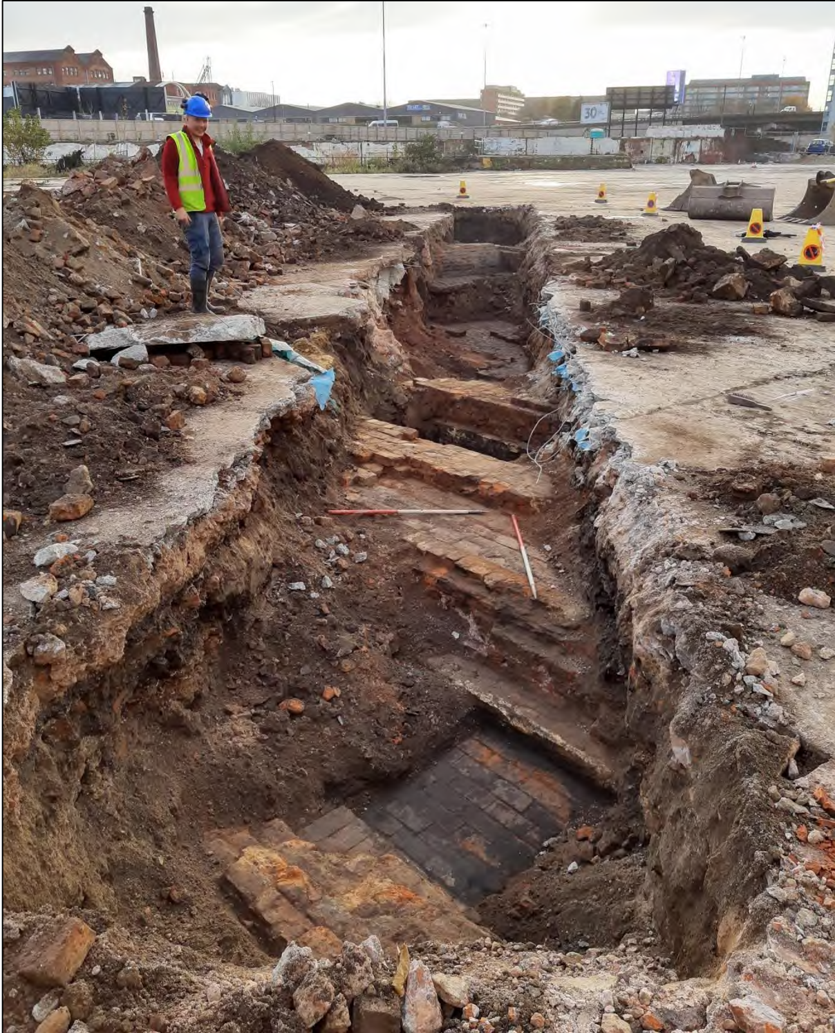
Plate 29: Trench 5, looking southwest.
