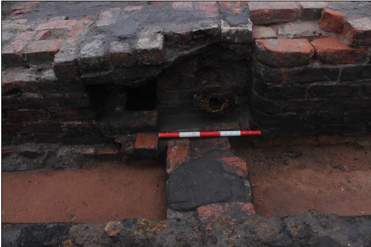
Plate 152: Wall 3189 and blocking 3191, together with 3070, looking west (0.50m scale)
