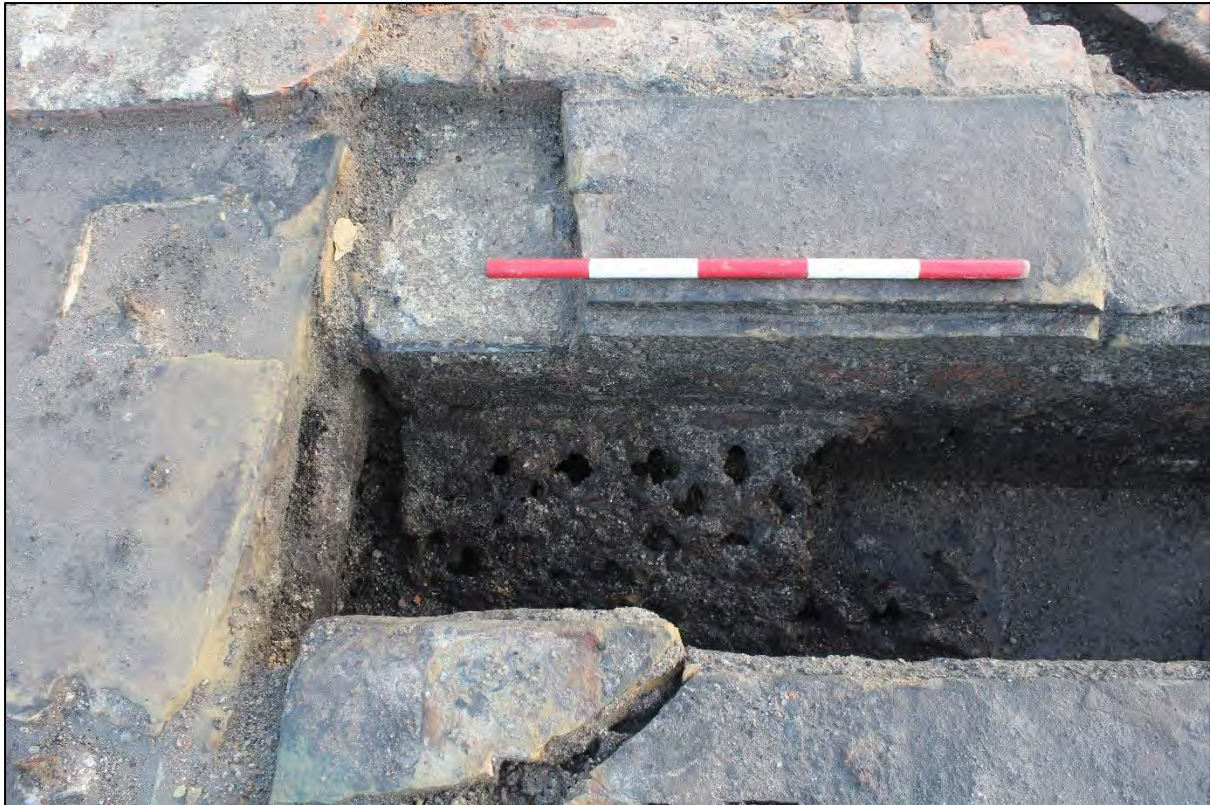
Plate 79: Detail of the drain interior, rebated stone coping and collapsed cast-iron grate
