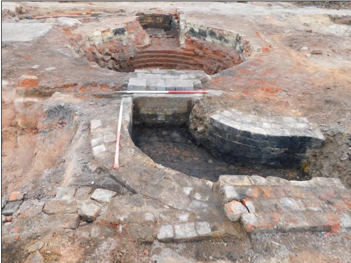
Plate 163: Flue 422 feeding into chimney 424 blocked by later brick wall 423, facing north (2 x 1m scales)
