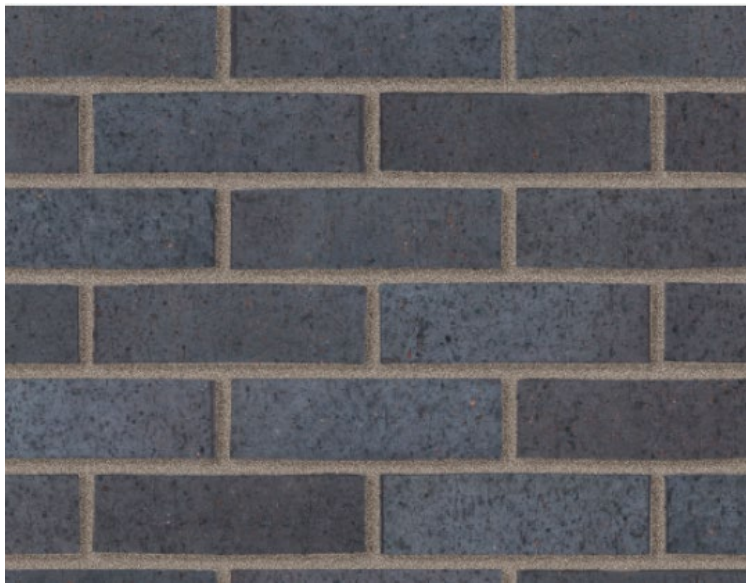
Brick Plinth -65mm Staffordshire Blue Dragfaced Engineering Bricks Sample sent 07.11.2025 to Sam Elliot and approved
