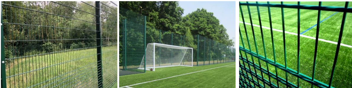
Rigid panel ballstop fencing to perimeter of facility, powder coated dark green to be discrete against a rural backdrop
