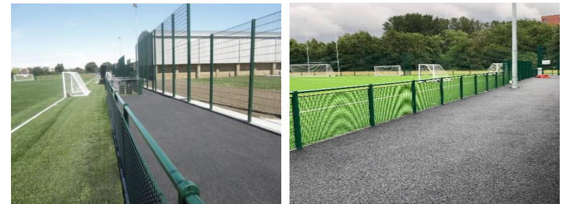
Porous macadam hardstanding to side of pitch
