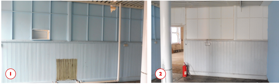
Original partitions to be carefully removed and kept for reuse by future tenants.
