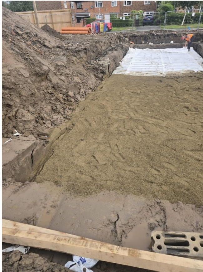
Photo 17: Backfill of cover above attenuation tank.
