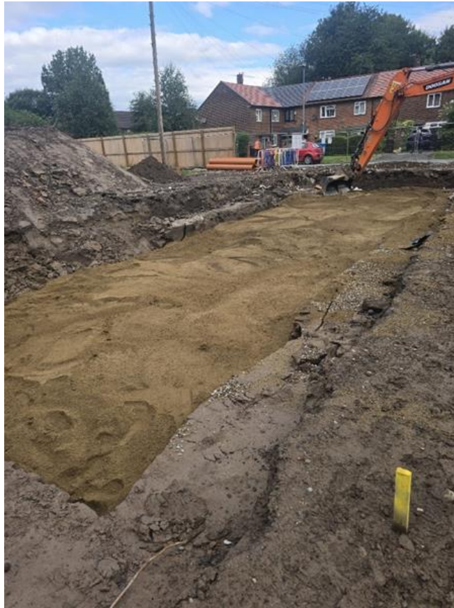
Photo 19: Backfill of cover above attenuation tank.
