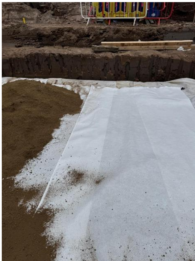
Photo 16: Installation of impermeable membrane over attenuation storage tank.
