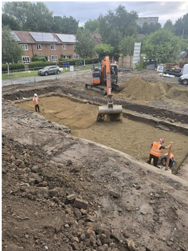
Photo 18: Backfill of cover above attenuation tank.
