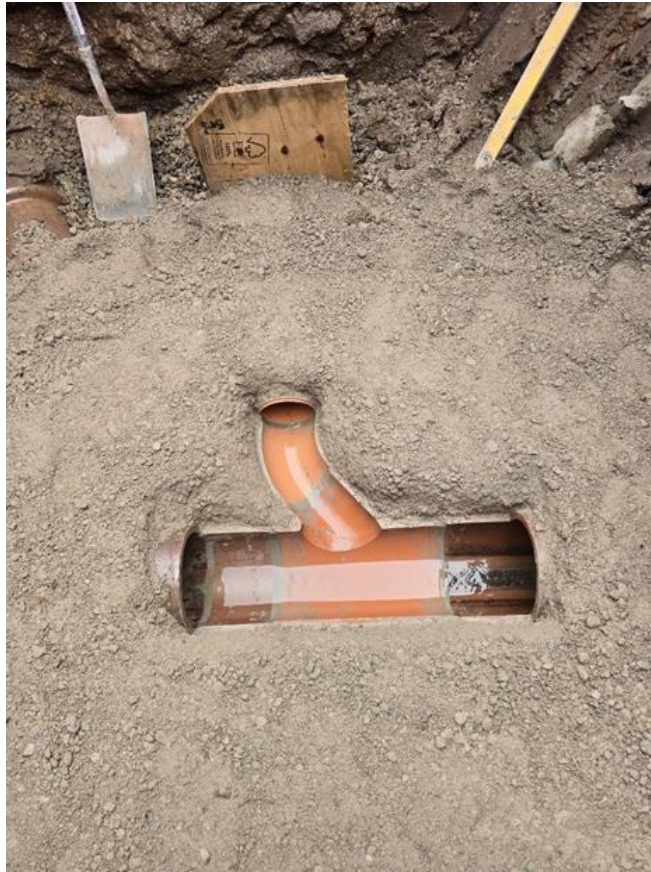
Photo 3: Angled pipe connection into existing UU sewer within Longhurst Road.
