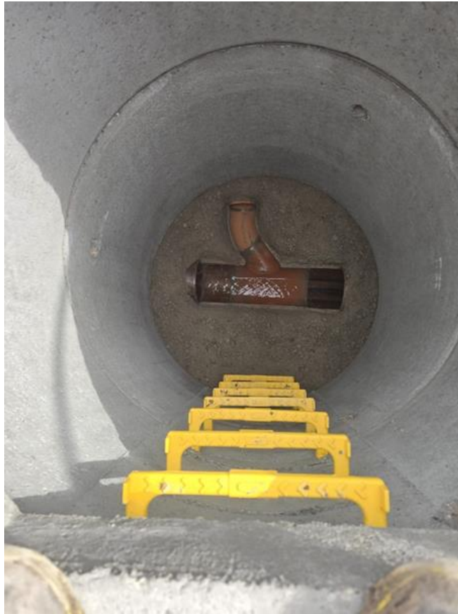
Photo 7: Angled pipe connection at base of new manhole within Longhurst Road after installation of manhole rings.
