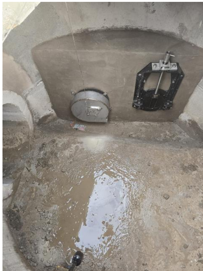
Photo 13: Installation of hydrobrake unit.
