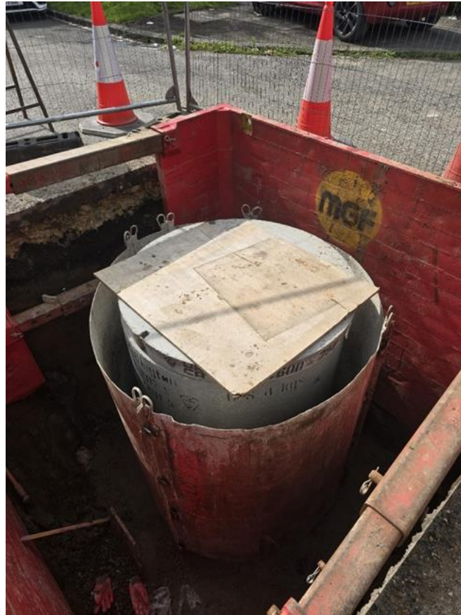
Photo 9: Installation of new manhole within Longhurst Road where connection into existing UU combined sewer will be located.
