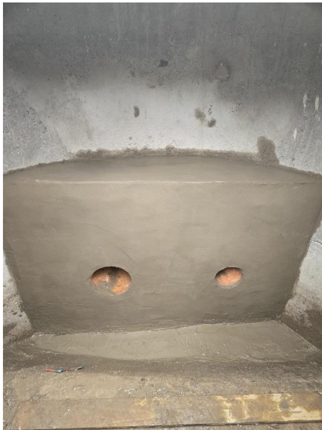
Photo 12: Casting of hydrobrake manhole benching ahead of hydrobrake installation.
