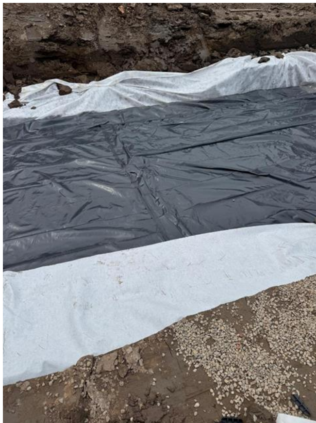
Photo 15: Installation of impermeable membrane over attenuation storage tank.
