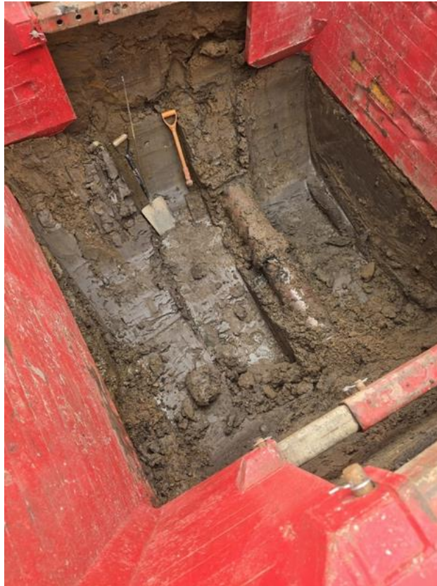
Photo 1: Excavation within Longhurst Road to expose existing UU combined sewer to install new connection.
