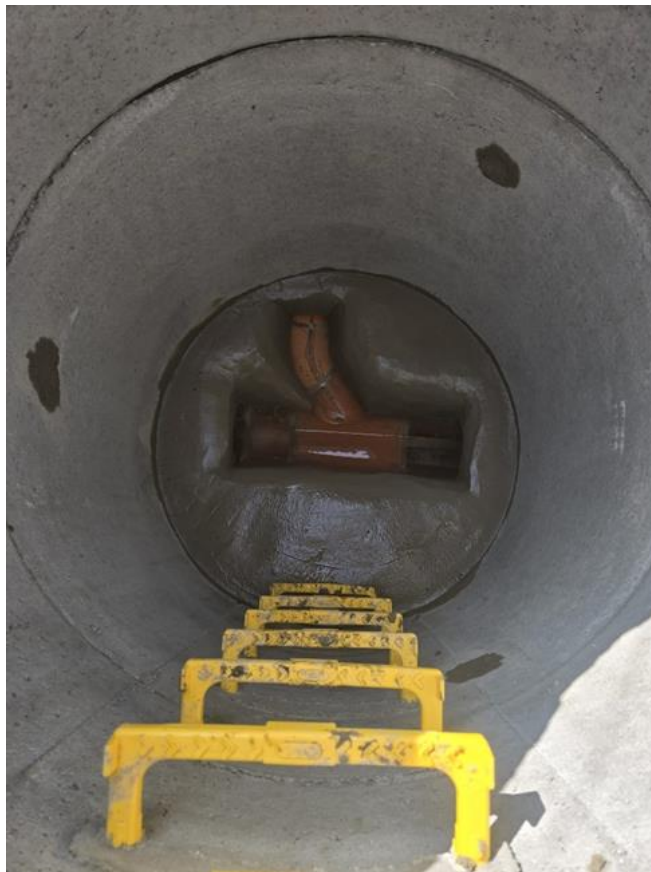
Photo 8: Concrete benching at base of new manhole within Longhurst Road after installation of manhole rings and new connection.
