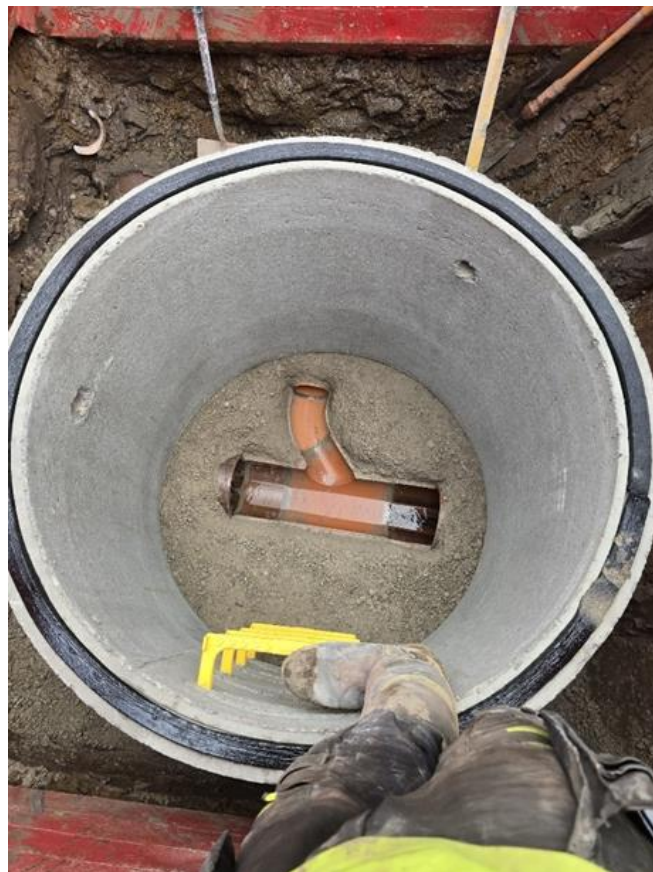
Photo 6: Angled pipe connection at base of new manhole within Longhurst Road after installation of manhole ring.
