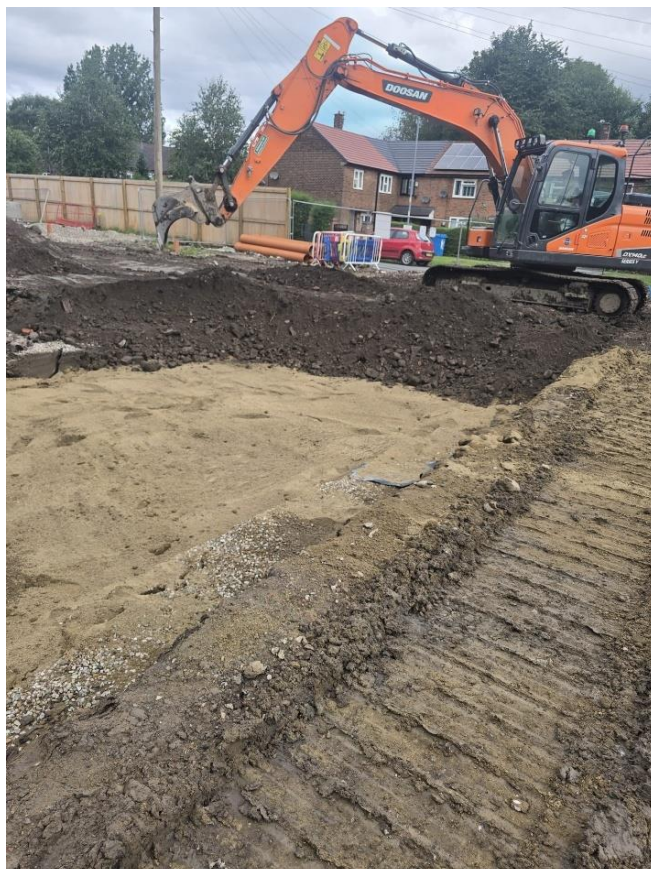
Photo 22: Backfill of cover above attenuation tank.
