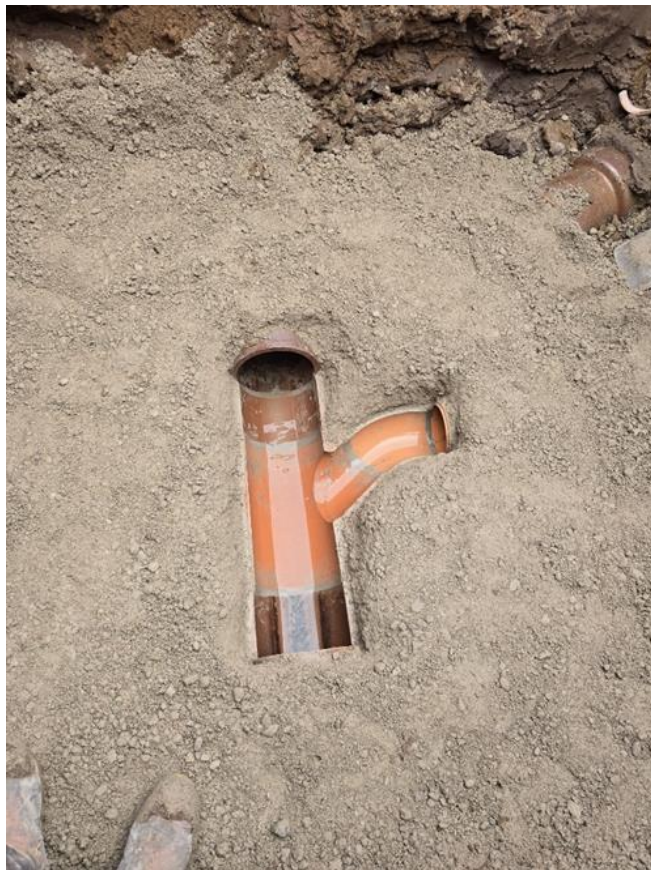
Photo 4: Angled pipe connection into existing UU sewer within Longhurst Road.
