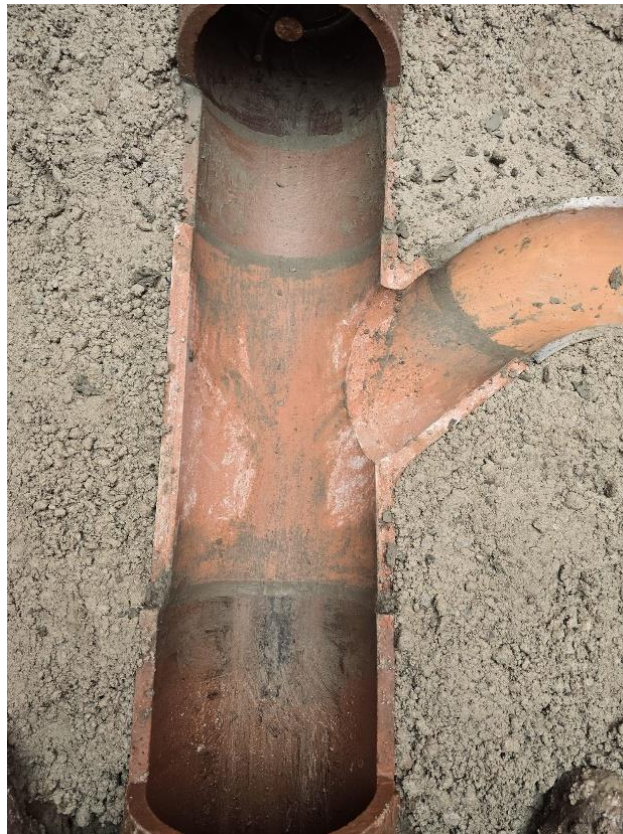
Photo 5: Angled pipe connection into existing UU sewer within Longhurst Road.
