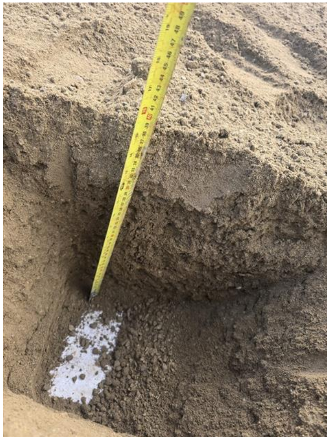
Photo 20: Depth of backfill above attenuation tank.
