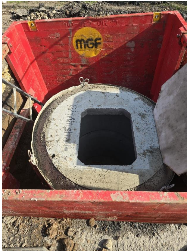
Photo 2: Installation of new manhole within Longhurst Road where connection into existing UU combined sewer will be located.
