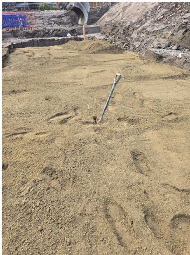
Photo 21: Backfill of cover above attenuation tank.
