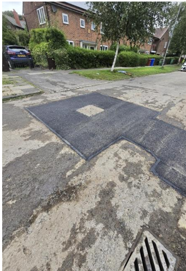
Photo 10: Finished ground and resurfacing surrounding new manhole connection into existing UU combined sewer within Longhurst Road.
