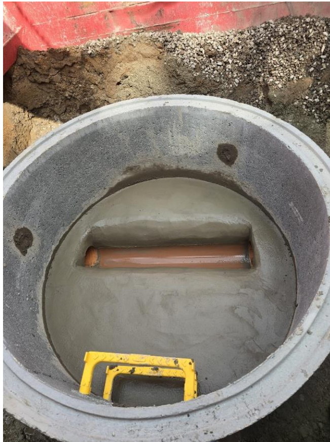
Photo 11: Casting of concrete manhole base along with first pre-cast manhole ring installation.
