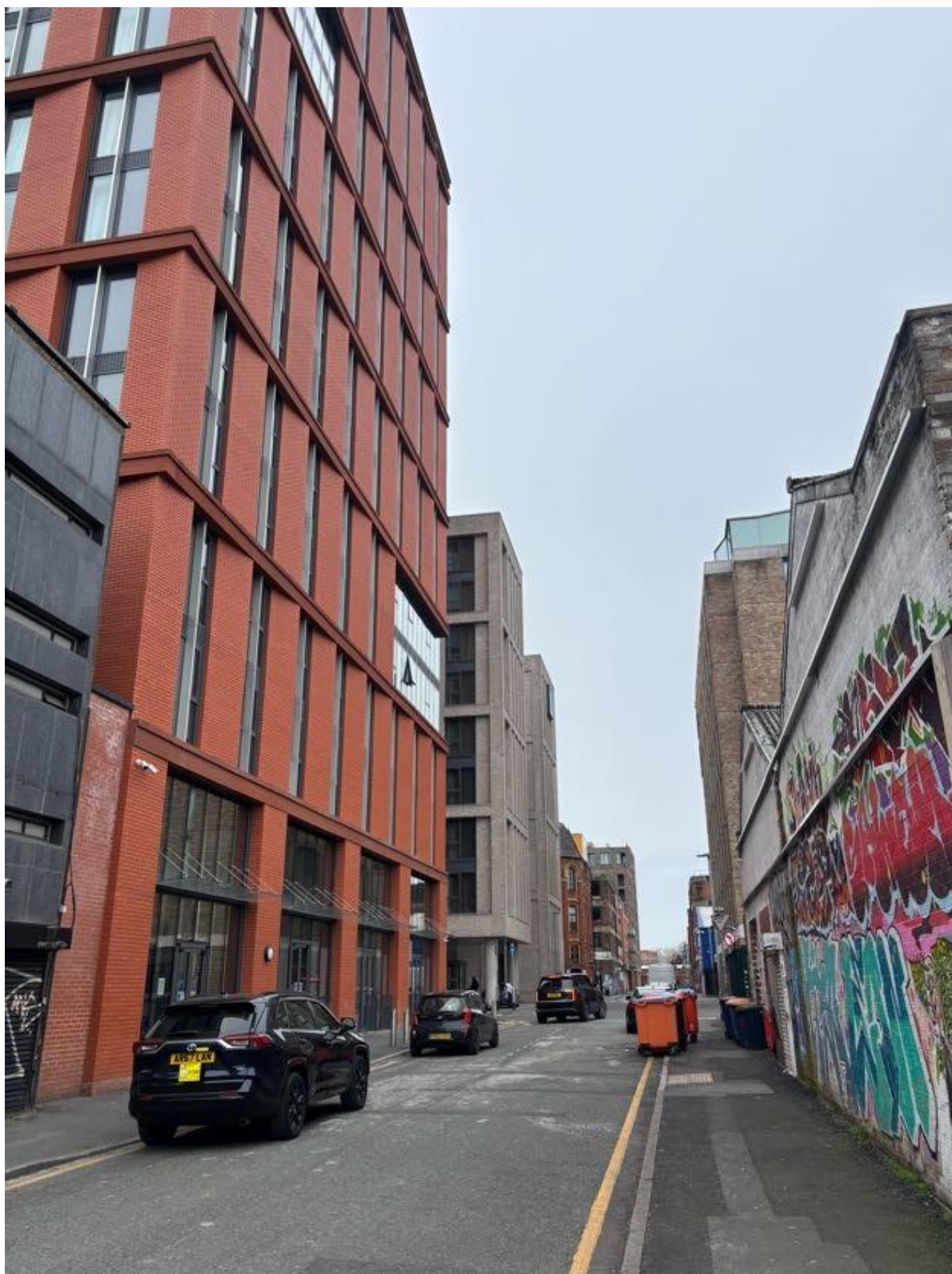
Photo 2: View from the edge of the Smithfield Conservation Area at the junction of Swan Street and Mason Street looking north along Mason Street towards the site.
