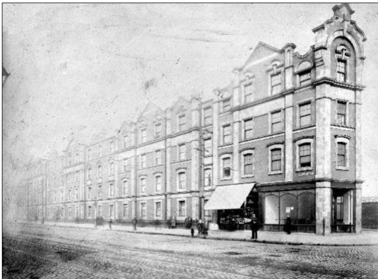
Alexandra Place at 18-20 Rochdale Road, 1906
