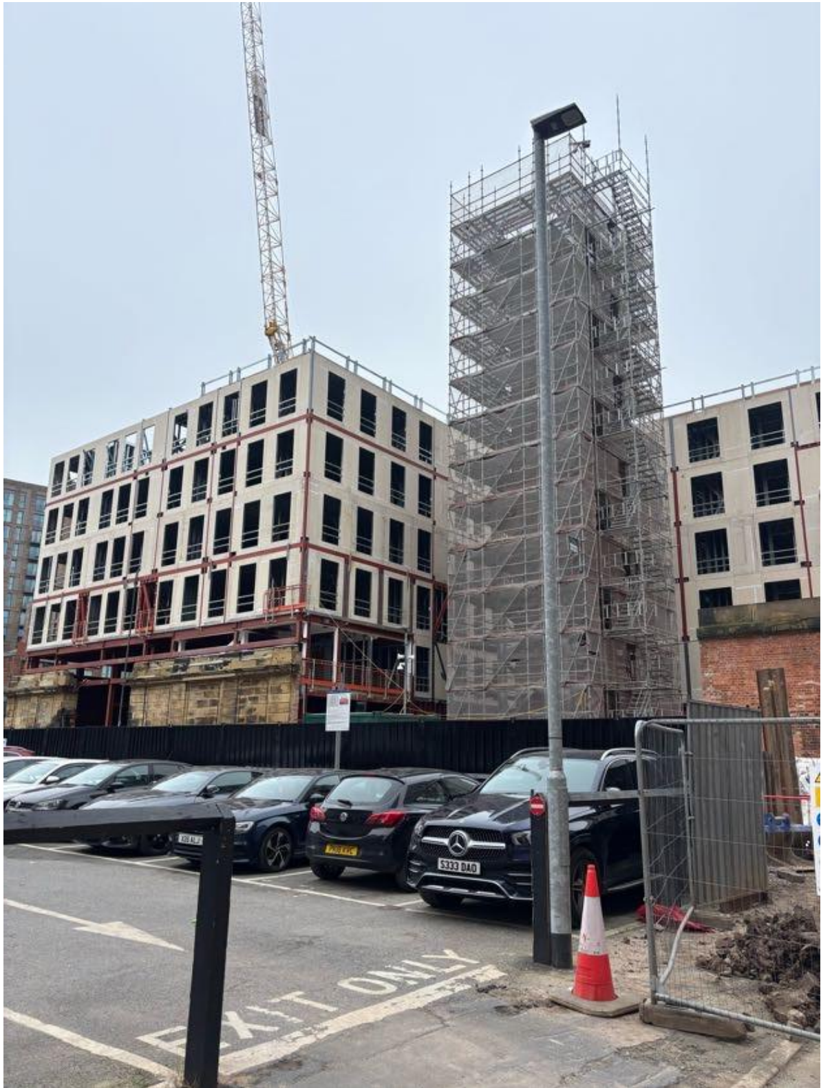
Photo 6: Viewpoint from the Former Police and Ambulance Station looking north-east towards the site.
