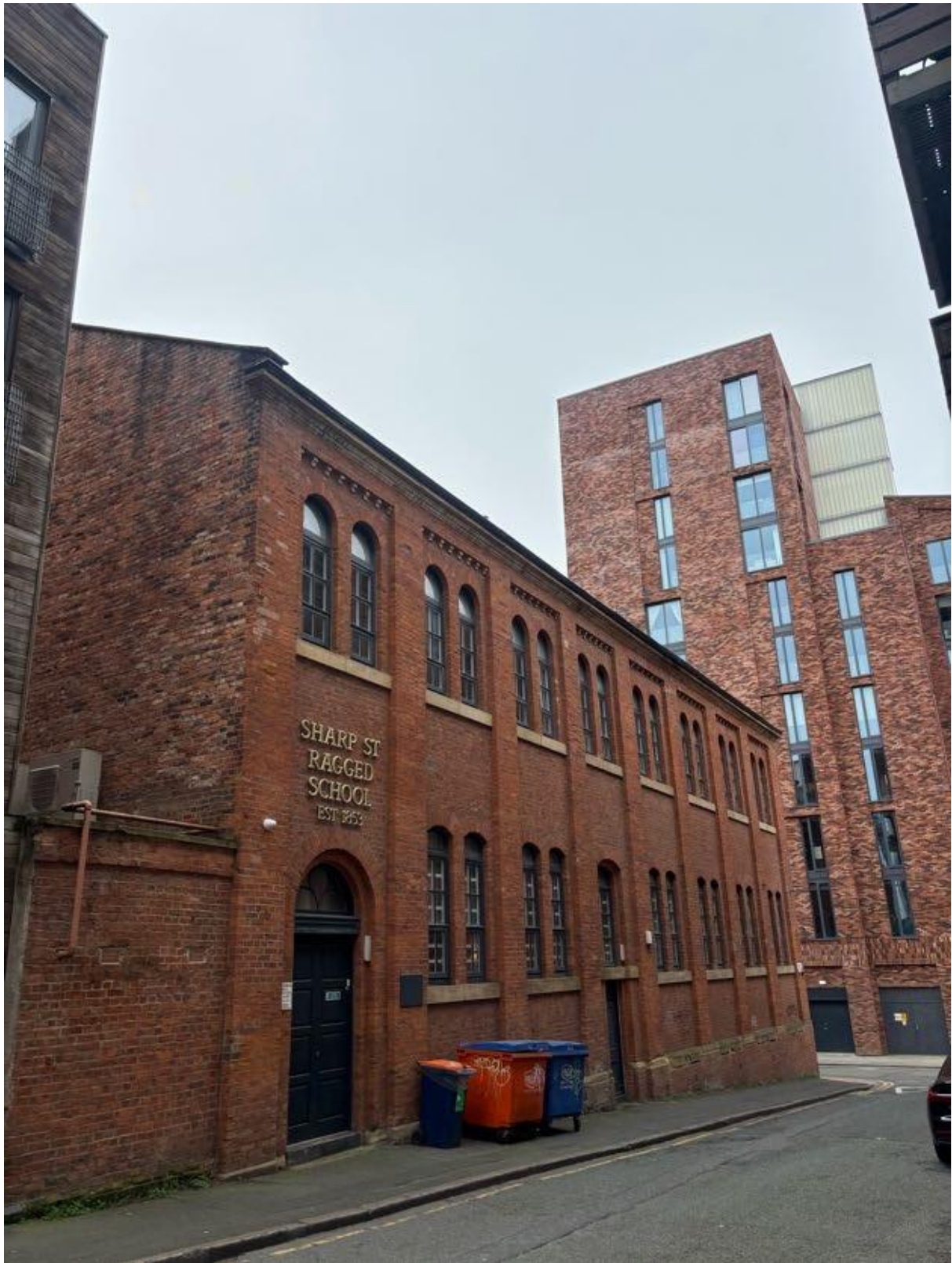
Photo 11: Sharp Street Ragged School, located along Sharp Street / Naples Street.
