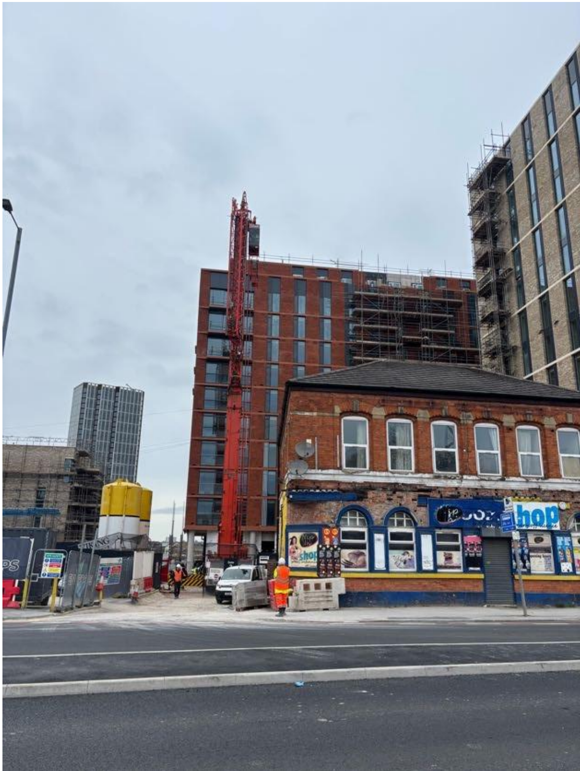
Photo 17: View of the site frontage along Rochdale Road, looking north-west.
