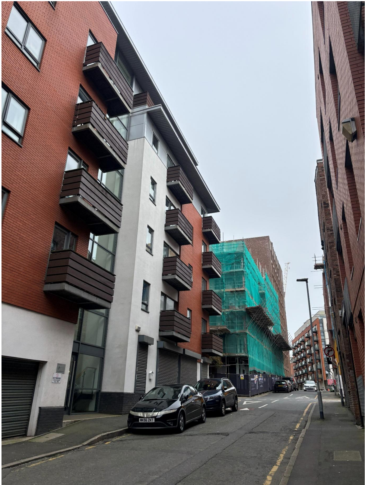
Photo 12: Viewpoint from Sharp Street Ragged School along Sharp Street, looking east towards the site.
