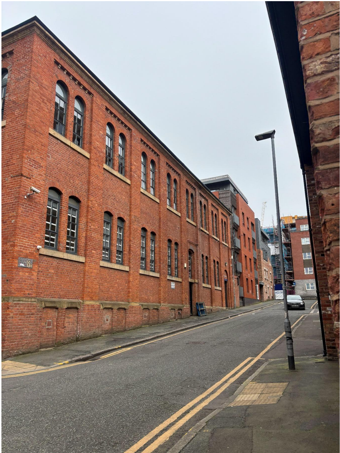
Photo 13: Viewpoint from Coop Printing Society along School Street, looking east towards the site.
