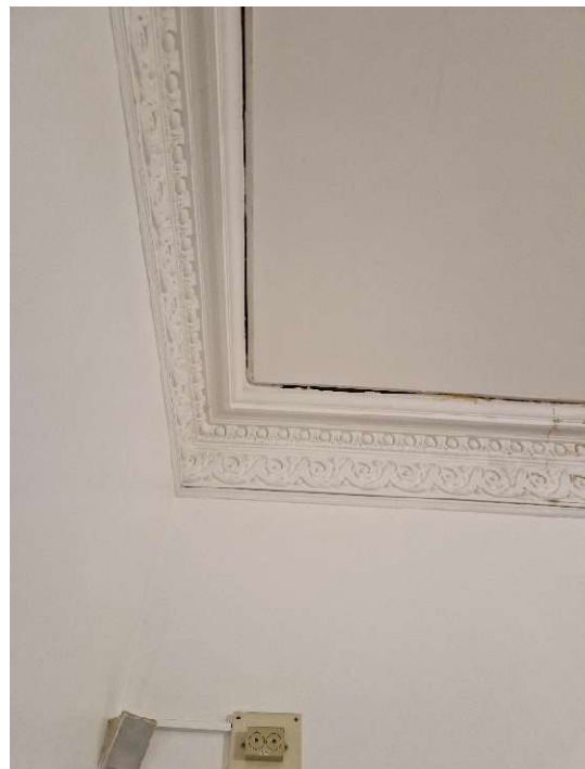
Photo 24 – Overboard to Lathe & Plaster Ceiling (Ground Floor)
