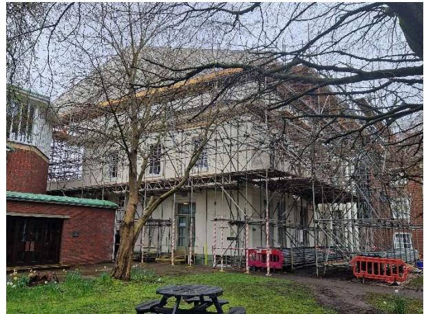
Photo 04 – Temporary Scaffold Roof to Rear Elevations
