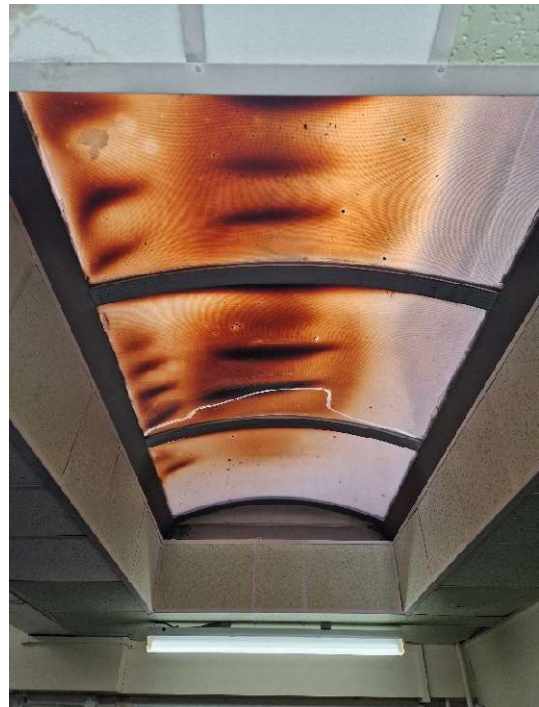
Photo 28 – Existing Rooflight (Ground Floor)
