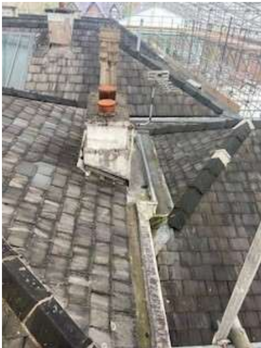
Photo 11 – Existing Roof Details
