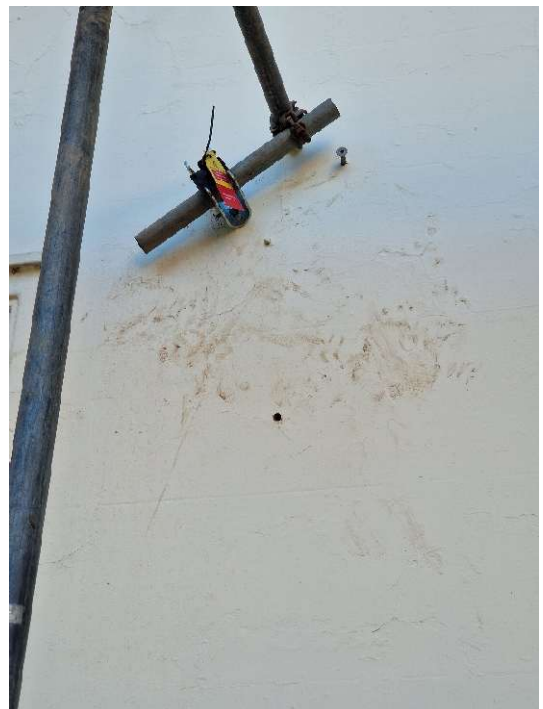
Photo 08 – Typical Scaffold Fixing
