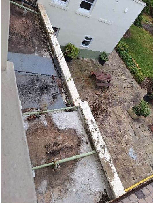
Photo 13 – Existing Flat Roof Covering (FR1)
