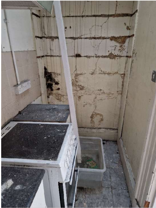
Photo 21 – Existing Kitchenette (First Floor)
