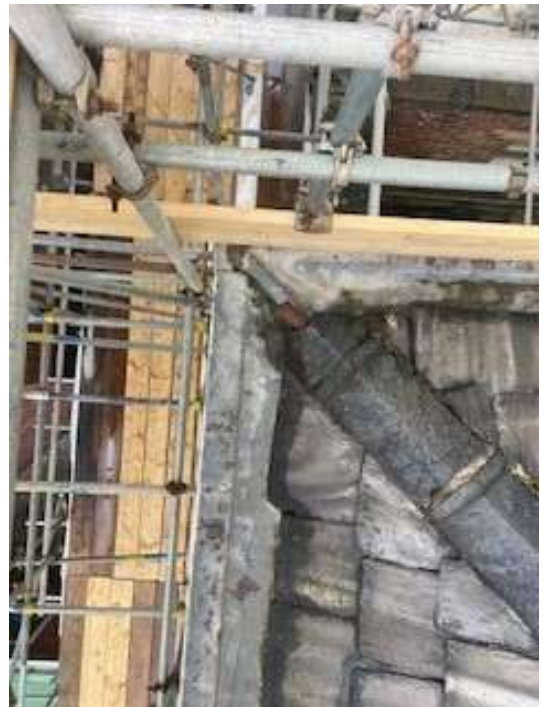
Photo 12 – Existing Gutter Details
