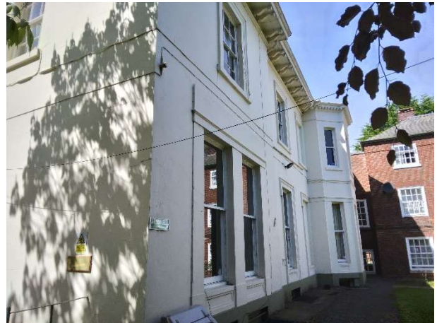
Photo 02 – Typical Side Elevation
