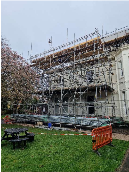
Photo 09 – Kentledge Scaffold to Rear Elevation
