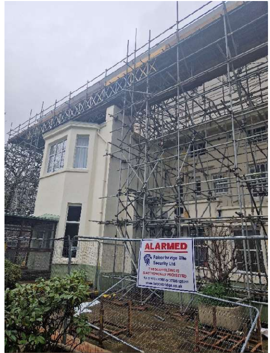
Photo 10 – Temporary Roof Scaffold to Side Elevation
