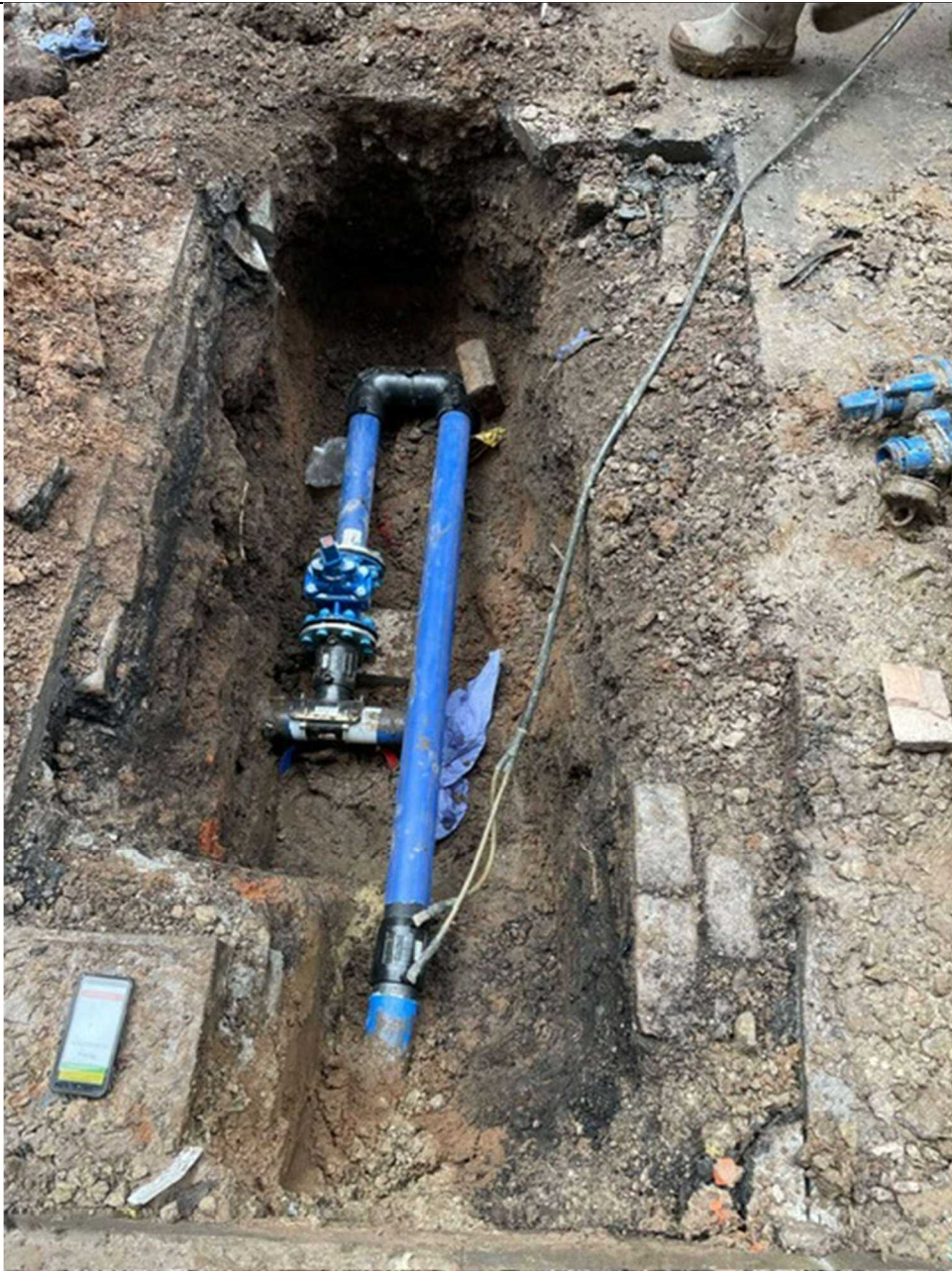
Photograph 1: Supply pipe installation.
