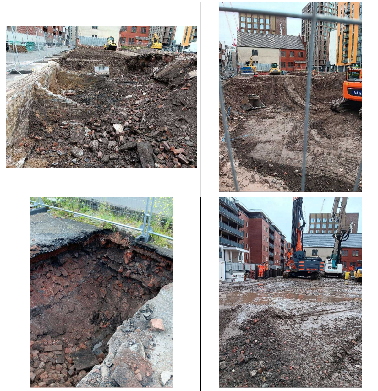
Plate 3-1: Photographs of groundworks at the site, including grubbing out of in-ground structures and piling operations.
