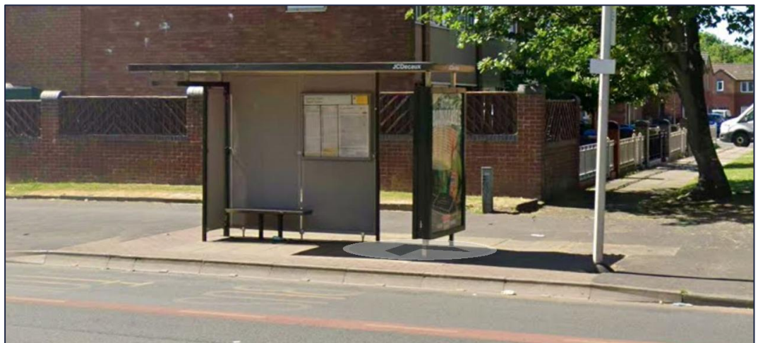
Figure 4.2 – Northbound Bus stop on Oldham Road
