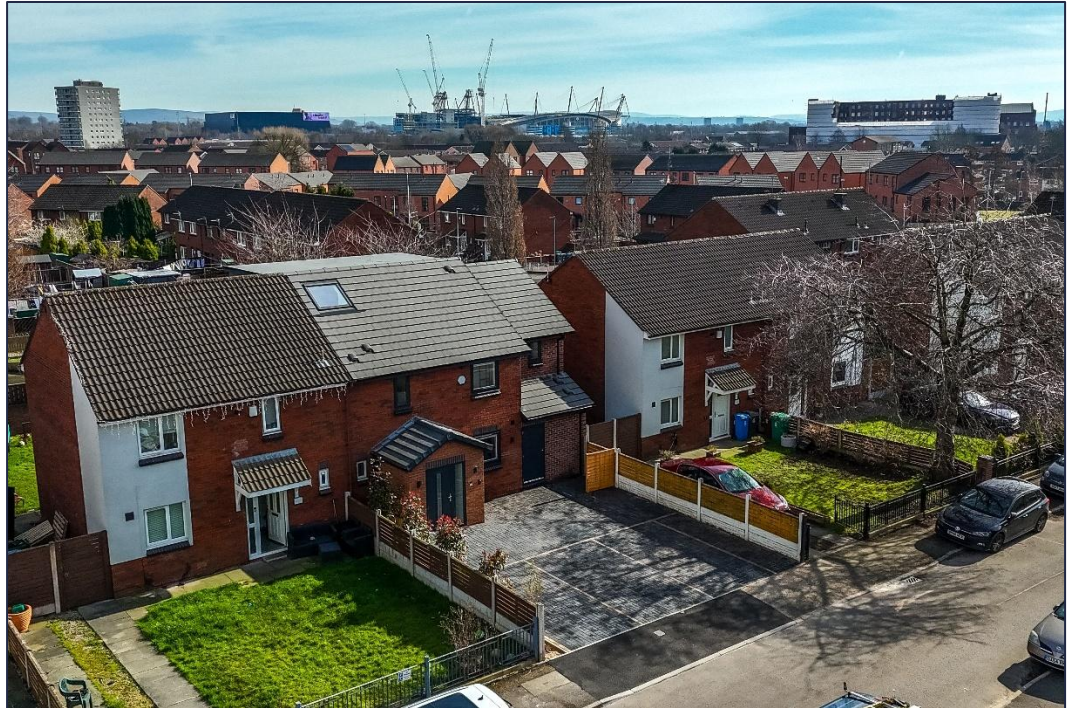
Figure 2.3 – General Aerial View of no.10 Landos Road
