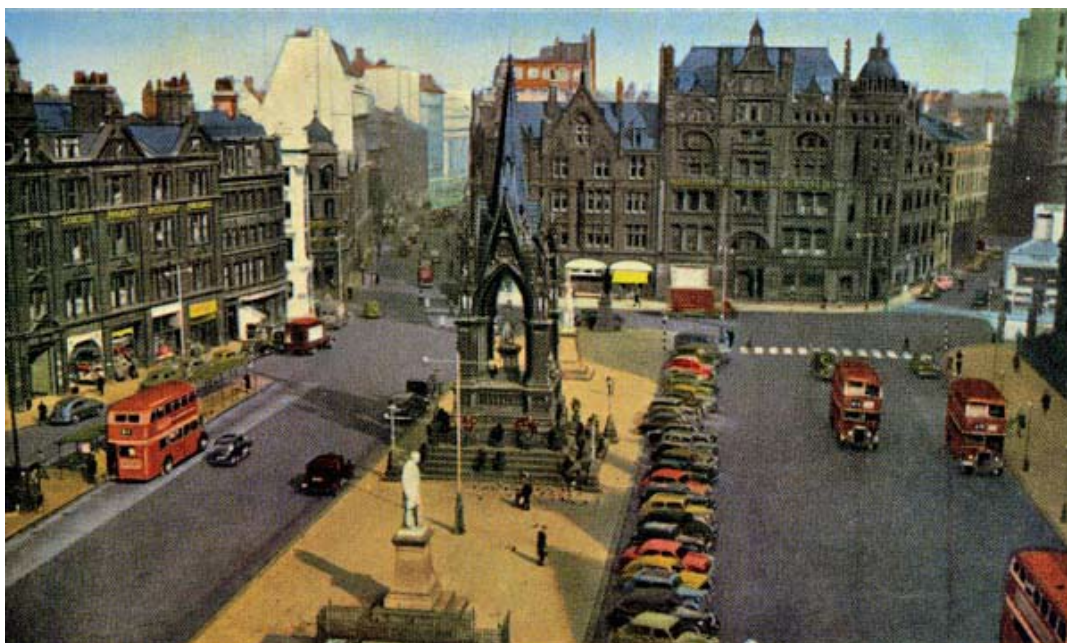
Fig 5: Mid-twentieth century postcard showing awnings to the shop fronts on Princess Street (centre).
