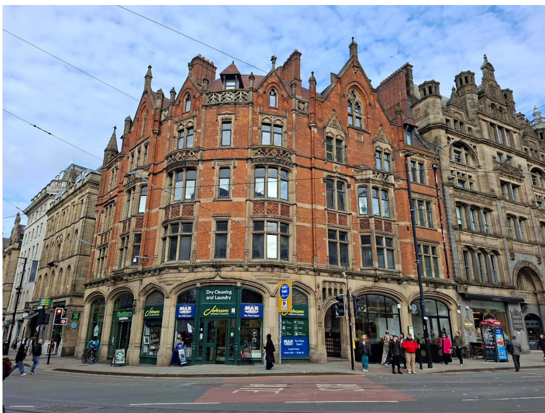
Fig 2: Close up view of 1-7 Princess Street (2-5 Princess Street is the two arched windows to centre-right of the image). The former Northern Assurance Building is to the right.
