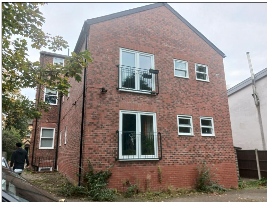
Figure 7.8: Photograph of as built extension.
