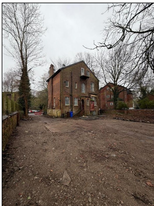
Figure 2.3: View towards building from the north east showing the rear elevation with 12 Deerpark Road in the background.
