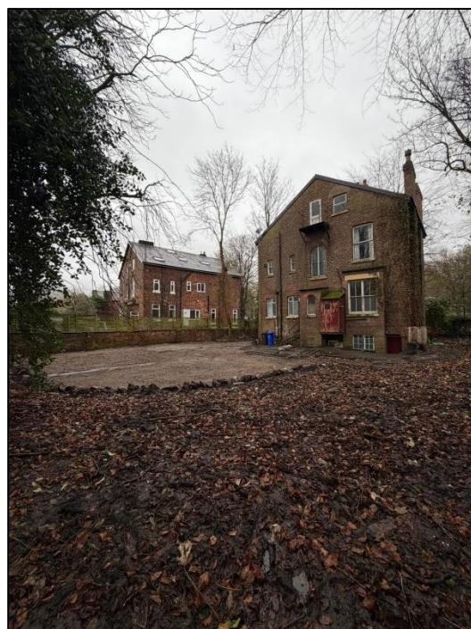
Figure 2.4: View towards building from the north west showing the rear elevation with 8 Deerpark Road in the background.
