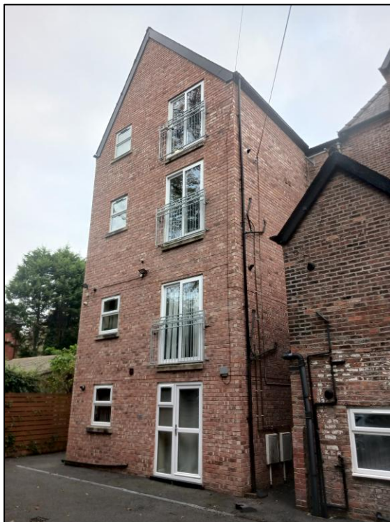
Figure 7.12: Photograph of as built four storey rear extension.
