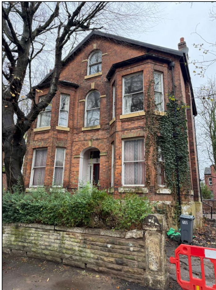
Figure 2.2: View of front elevation.
