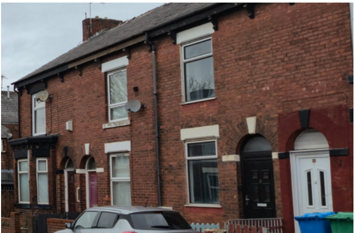
Expressed lintels Contrasting masonry lintels are expressed on the façades of the terraced housing. Rainwater pipes also serve to break up the long blocks - typically every other house.
