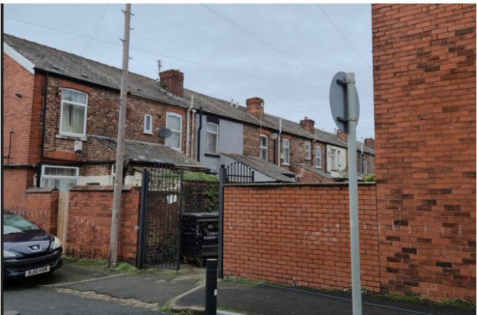
Boundary Single storey brick walls surround the yards to each terraced house. At the end of the terrace is a gate providing shared access to the rear of the properties.
