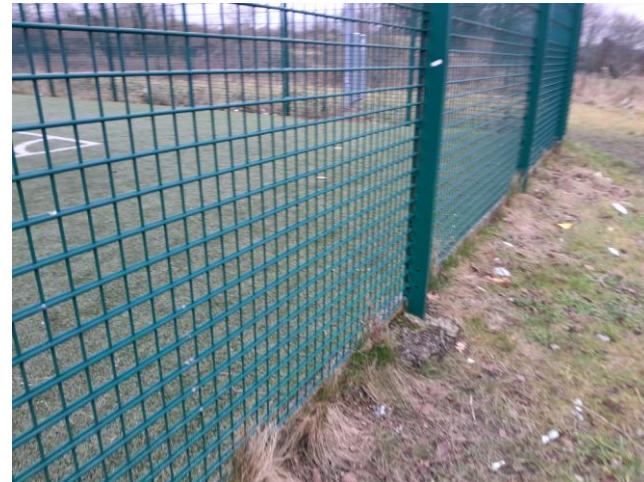
Photo 4: Developed land; sealed surface - the existing astroturf field.
