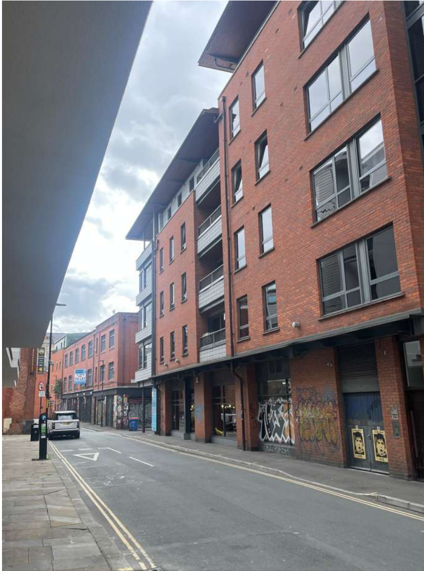
View from junction of High Street and Copperas Street
