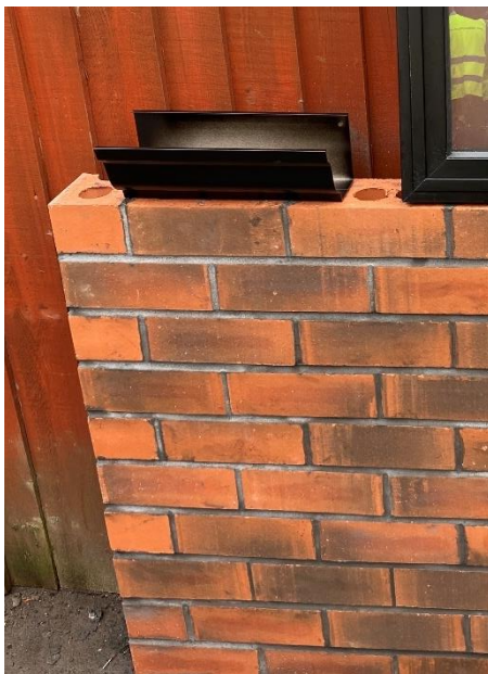
Figure 3: Sample on site with brick sample
