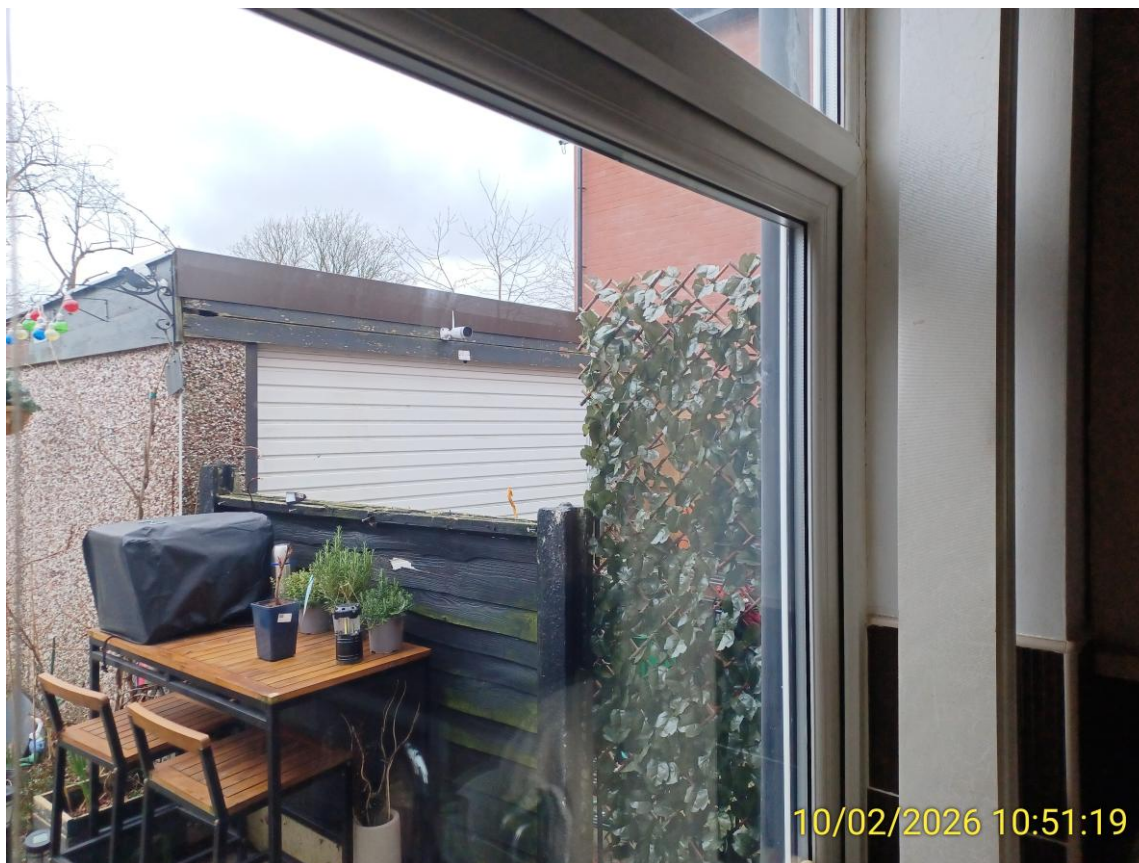
Photograph 5 Case officer site photograph of the kitchen window at no.34 Hawthorn Road, taken on the date shown.
