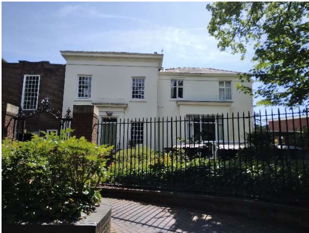
Photo 01 – Existing Front Elevation
