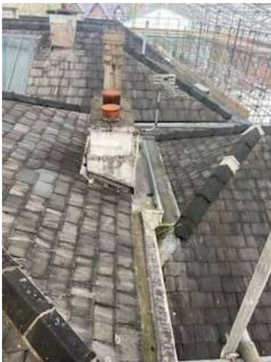
Photo 11 – Existing Roof Details
