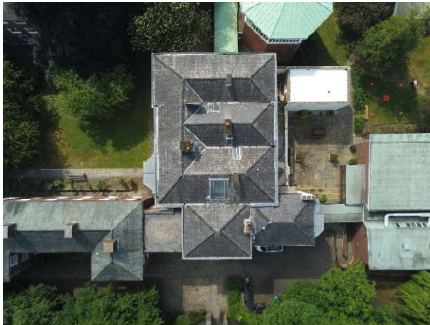
Photo 03 – Aerial Roof View
