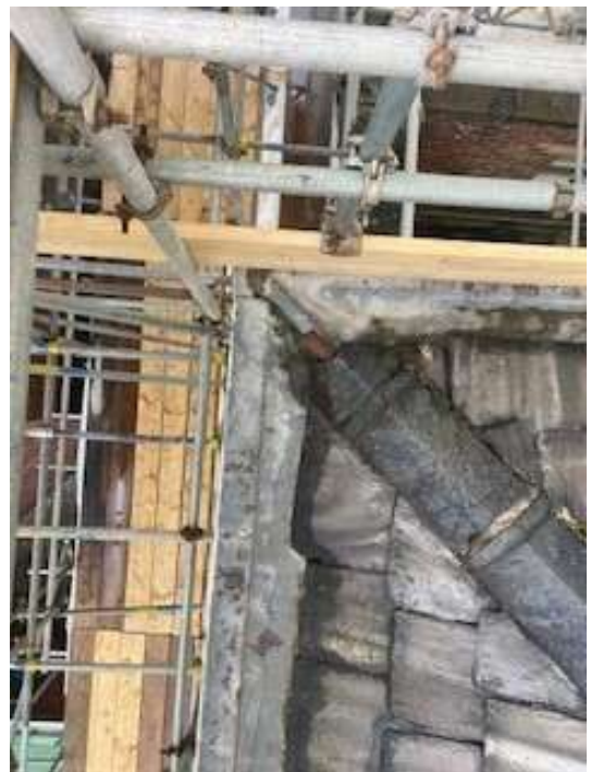
Photo 12 – Existing Gutter Details
