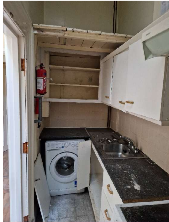
Photo 22 – Existing Kitchenette (First Floor)
