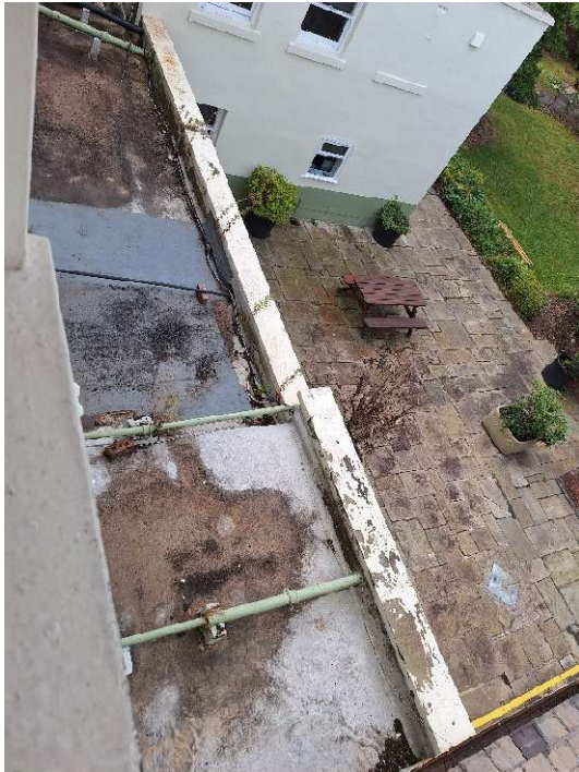
Photo 13 – Existing Flat Roof Covering (FR1)
