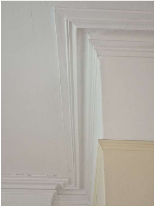
Photo 25 – Typical Ceiling Articulation
