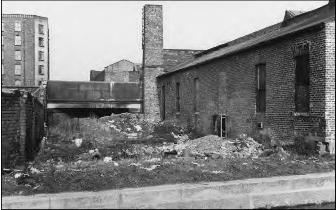
Plate 19: View of Jersey Street bridge during infilling, 1972, courtesy of Manchester Local Image Collection
