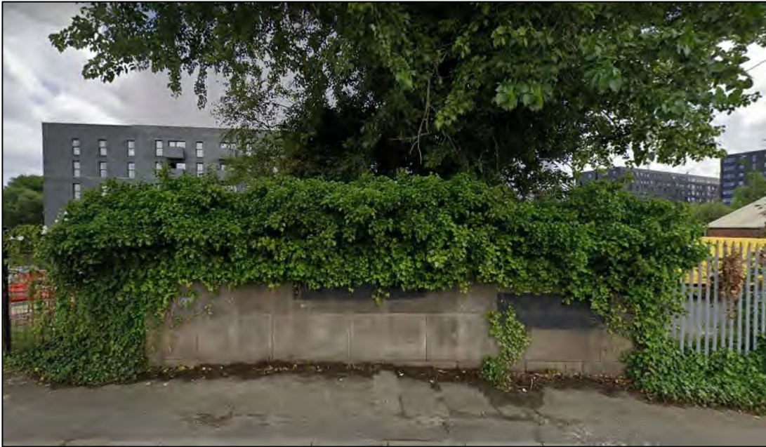
Plate 17: Canal bridge within the Site boundary at Jersey Street
