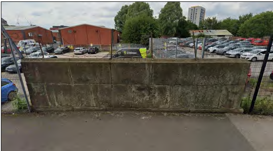
Plate 18: Canal bridge within the Site boundary at Jersey Street
