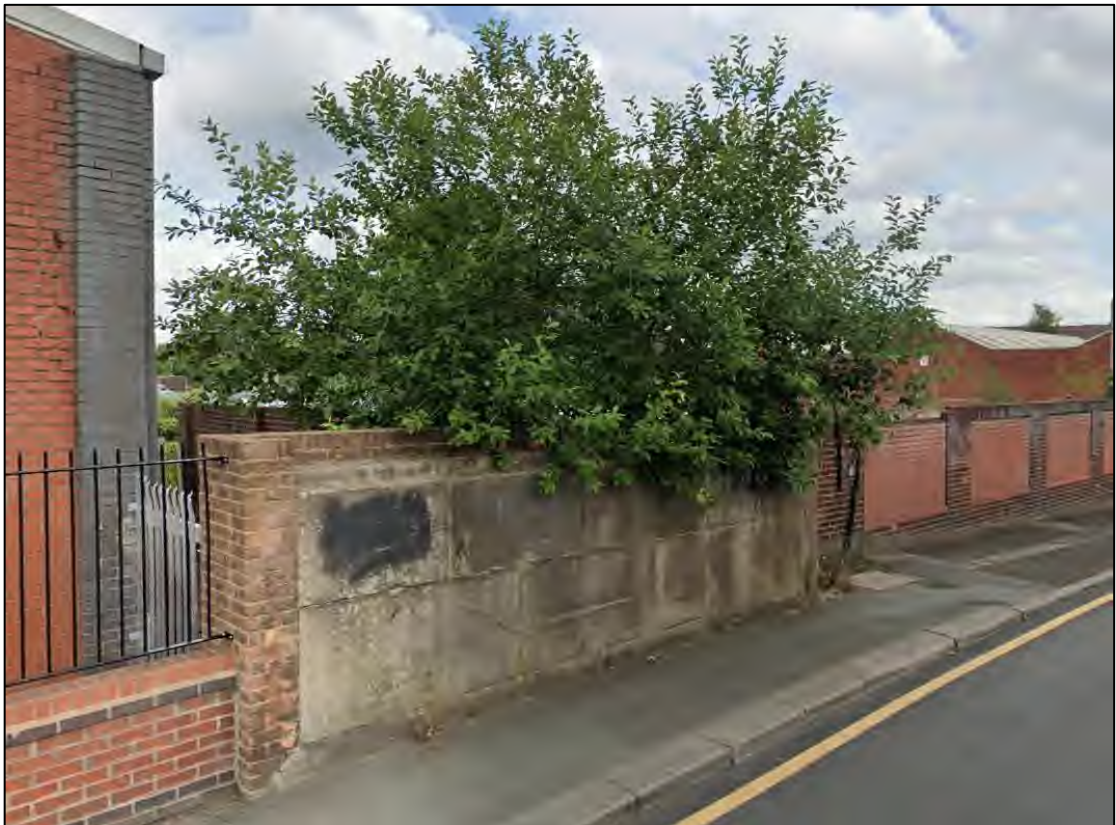
Plate 20: Canal bridge within the Site boundary at Poland Street
