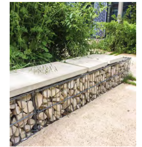
Precedent image: Gabion Wall which forms part of Mobility Hub development
