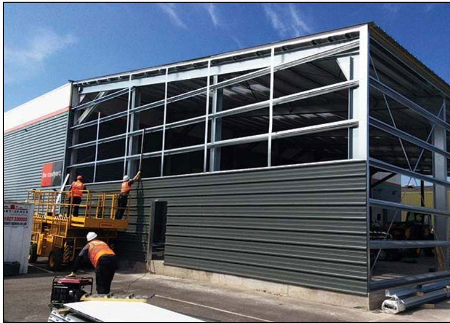
Fig 9: External Cladding Installation
