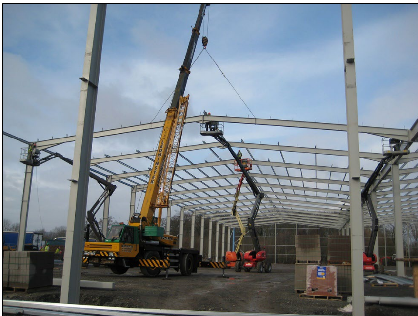
Fig 8: Structural Steel Frame erected using Mobile Crane & MEWPS
