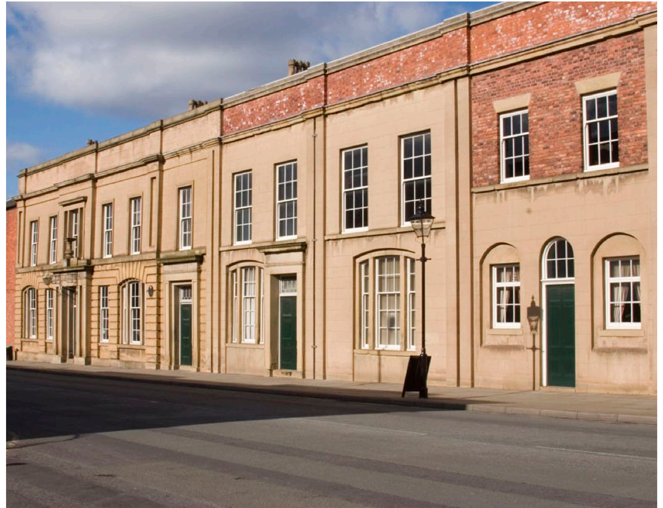
Image 25 : Recent view of Liverpool Road elevation, showing Station Buildings.
