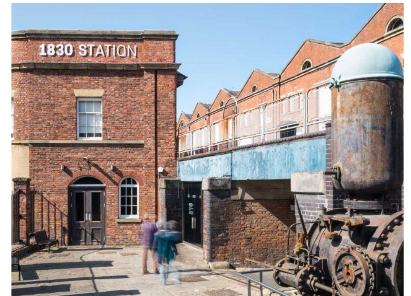
Image 3: 1830 Station Building in its current form, with railway alongside and 1830 Warehouse to right hand side of image. SIM website.
