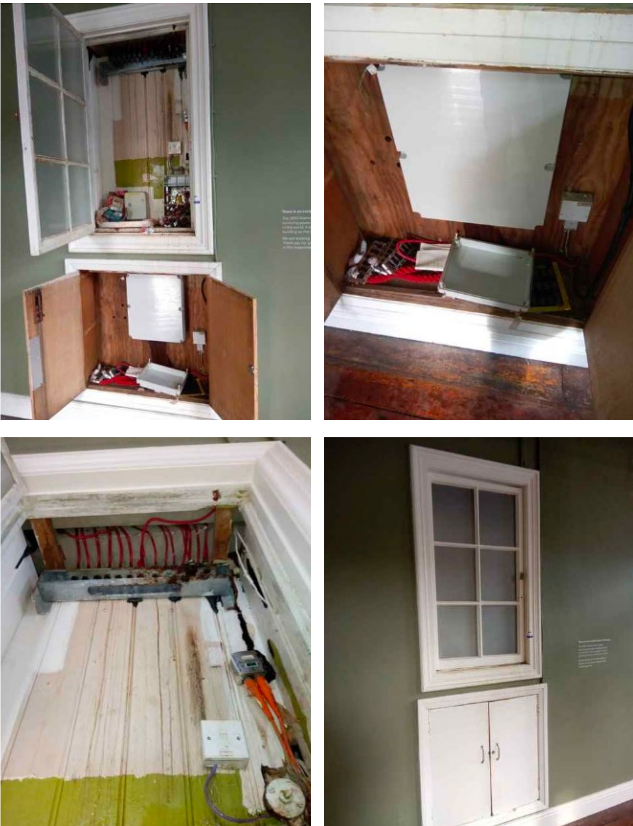
Images 13, 14, 15, 16, showing cupboard to location 0031:38, to be relined.
