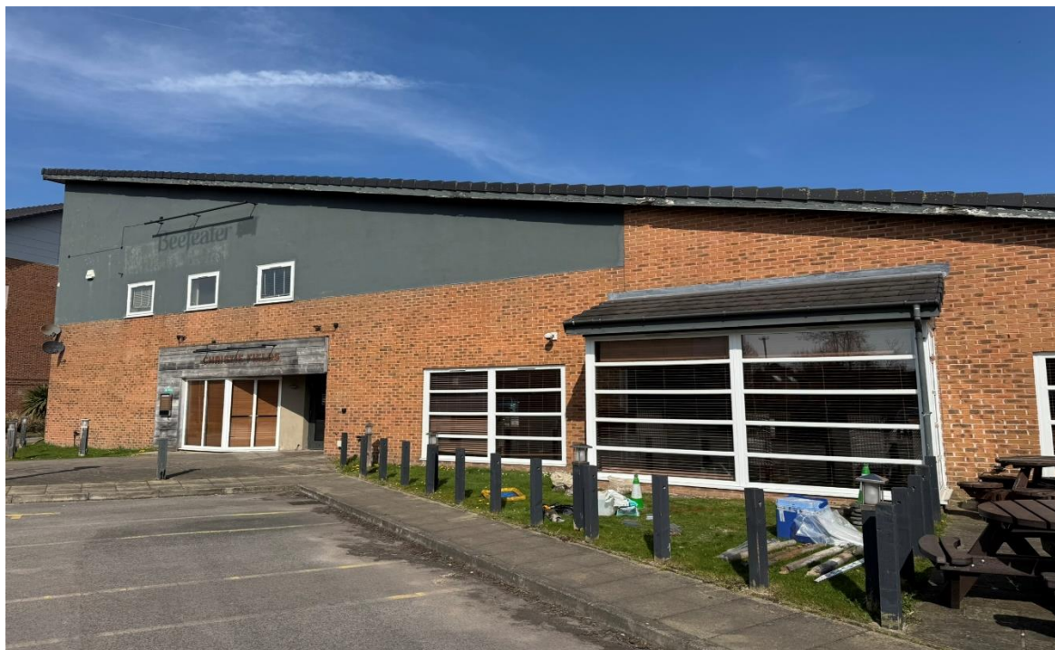
Plate 4 – Existing Brewers Fayre Looking North
