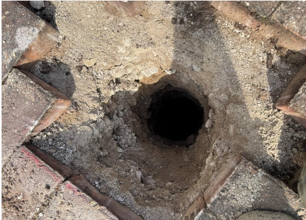
Plate 5 – WS02, GL to 0.60m bgl Pavement.
