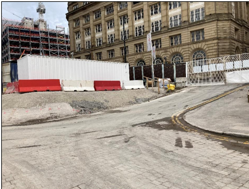
Photograph 1 showing the bare ground
