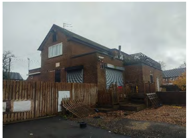
Figure 12 – The former nursery building as seen from the northern site section, looking south-west.
