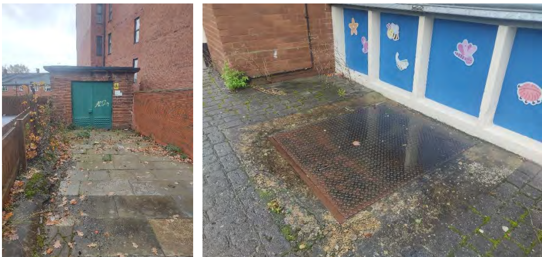
Figure 8: An off-site electricity substation adjacent to the eastern site boundary (left) and a metal cover of historical beer storage when the site was utilised as a public house (right).
