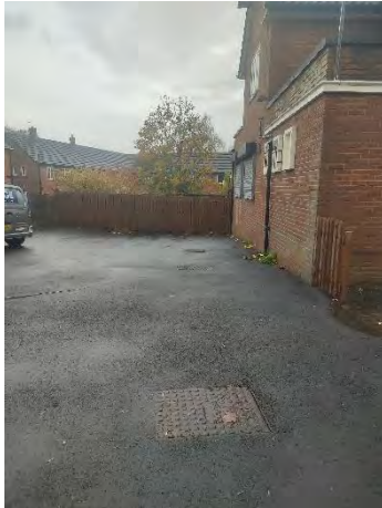
Figure 3 – Manholes in the western car park, looking north.
