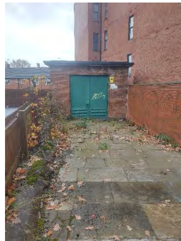
Figure 20 – The off-site electrical substation by the eastern site boundary, looking north.
