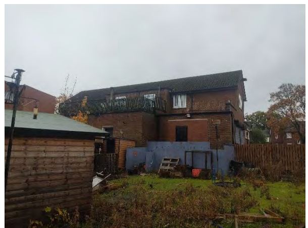
Figure 6 – The northern site section, looking south-east.
