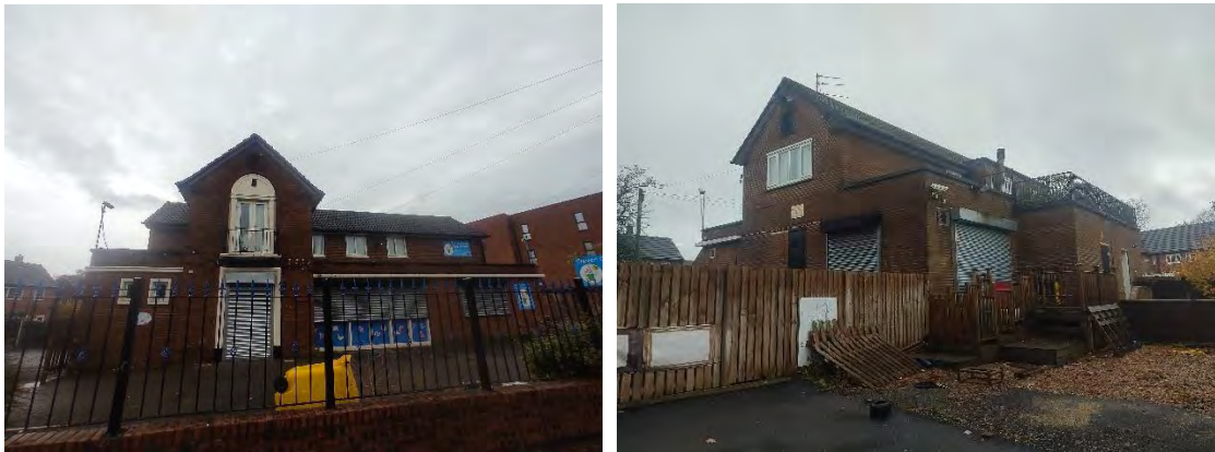
Figure 5: The former Clever Clowns Nursery as seen from the southern site section, looking north (left) and from the northern site section comprising former play areas, looking south-west (right).
