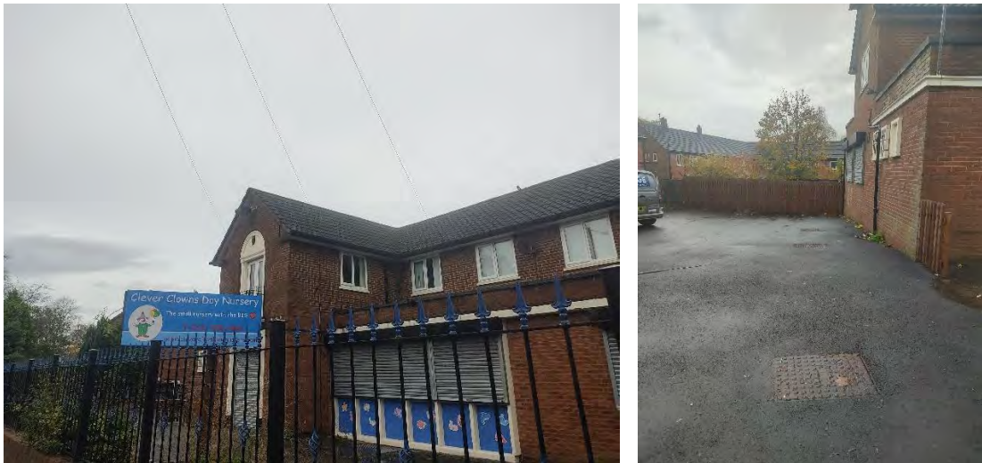
Figure 7: The overhead BT / electric cables connecting to site in the southern section (left) and manholes in the western site section – car park (right).
