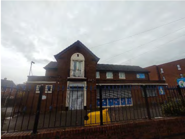
Figure 1 – The nursery building and the southern site section, looking north.
