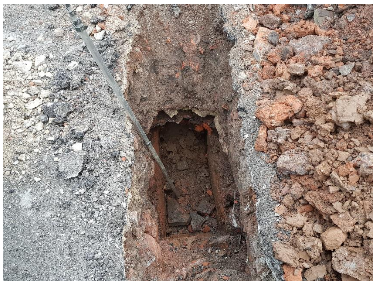
TP104: Internal view of excavation.
