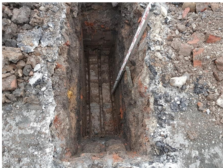
TP101: Internal view of excavation.
