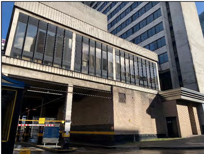
Photo 3 Concrete construction of building
