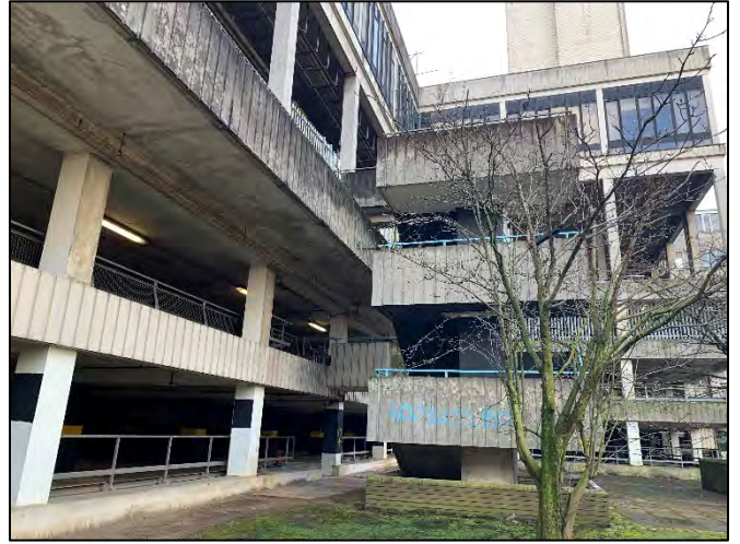
Photo 10 Open face multi-storey car park facing onto the River Irwell
