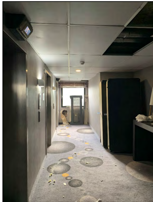
Photo 12 Example of internal aspect of the structure
