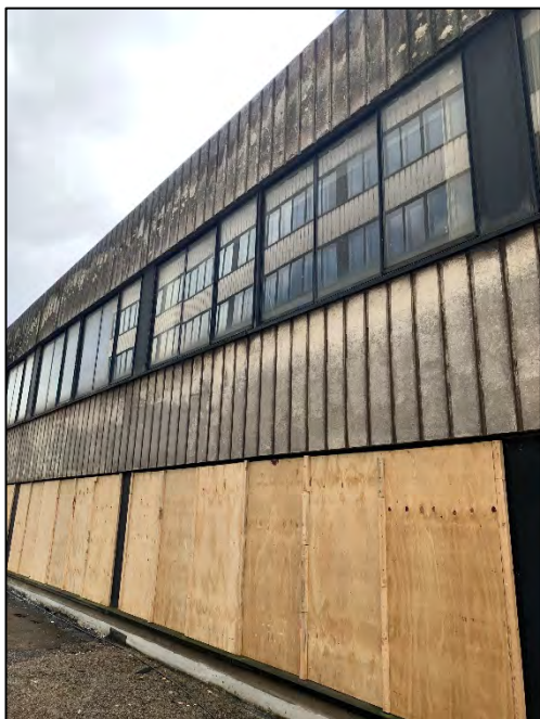
Photo 5 The back of Premier House (north face) with wooden boarding
