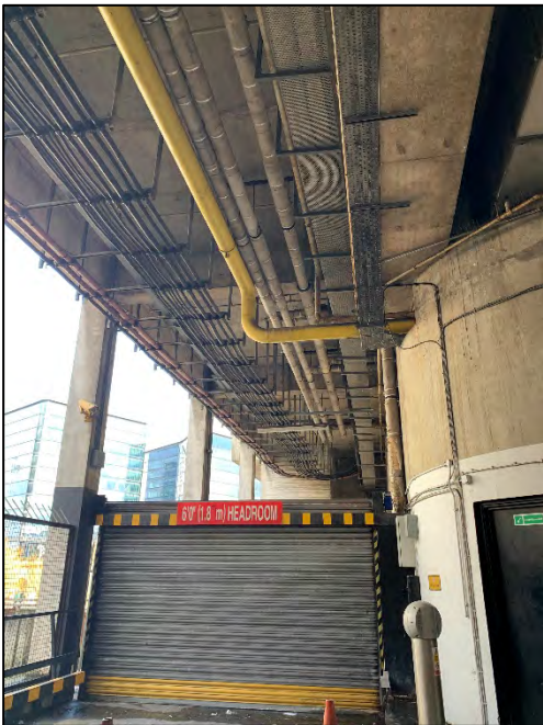
Photo 11 Example of service yard construction
