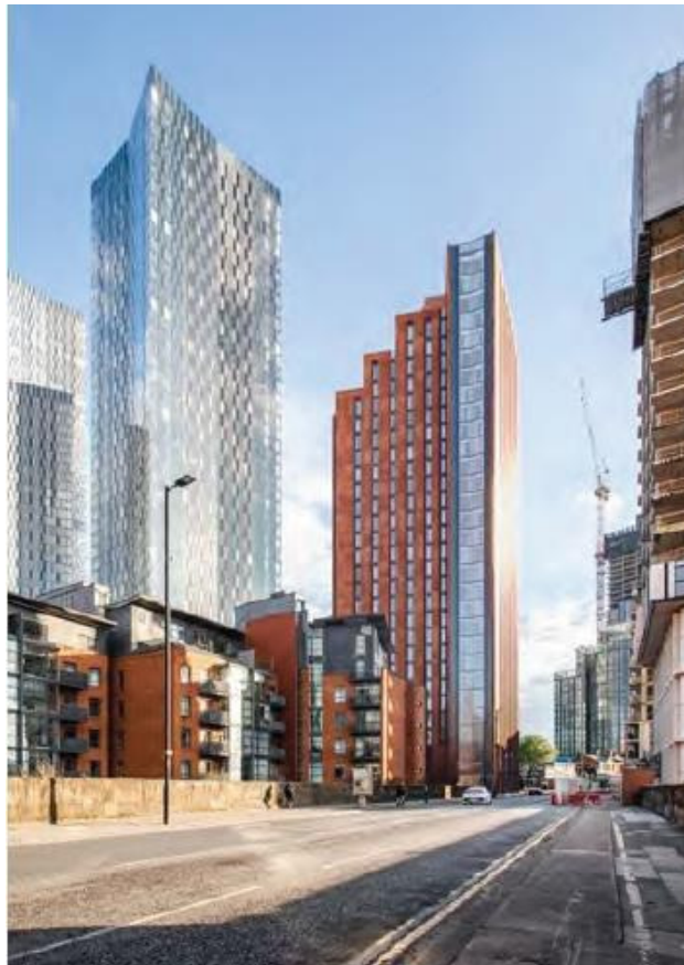
View from North-Eastern approach along Bridgewater Viaduct
