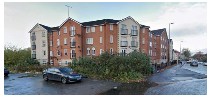
Apartment block further along Elizabeth Street
