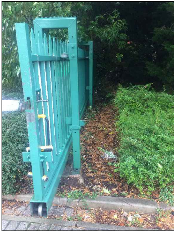
Existing Sliding Vehicular Barrier: To be removed
