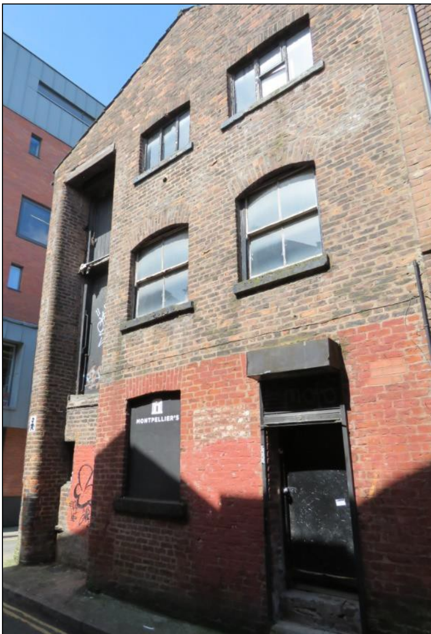
Figure 4. 7 Kelvin Street (2016) showing the brick gable to cleaned and restored.
