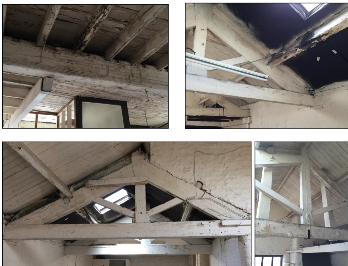
Figure 10 Details of the exposed roof timbers (May 2016). Further detailed surveys have been completed.
