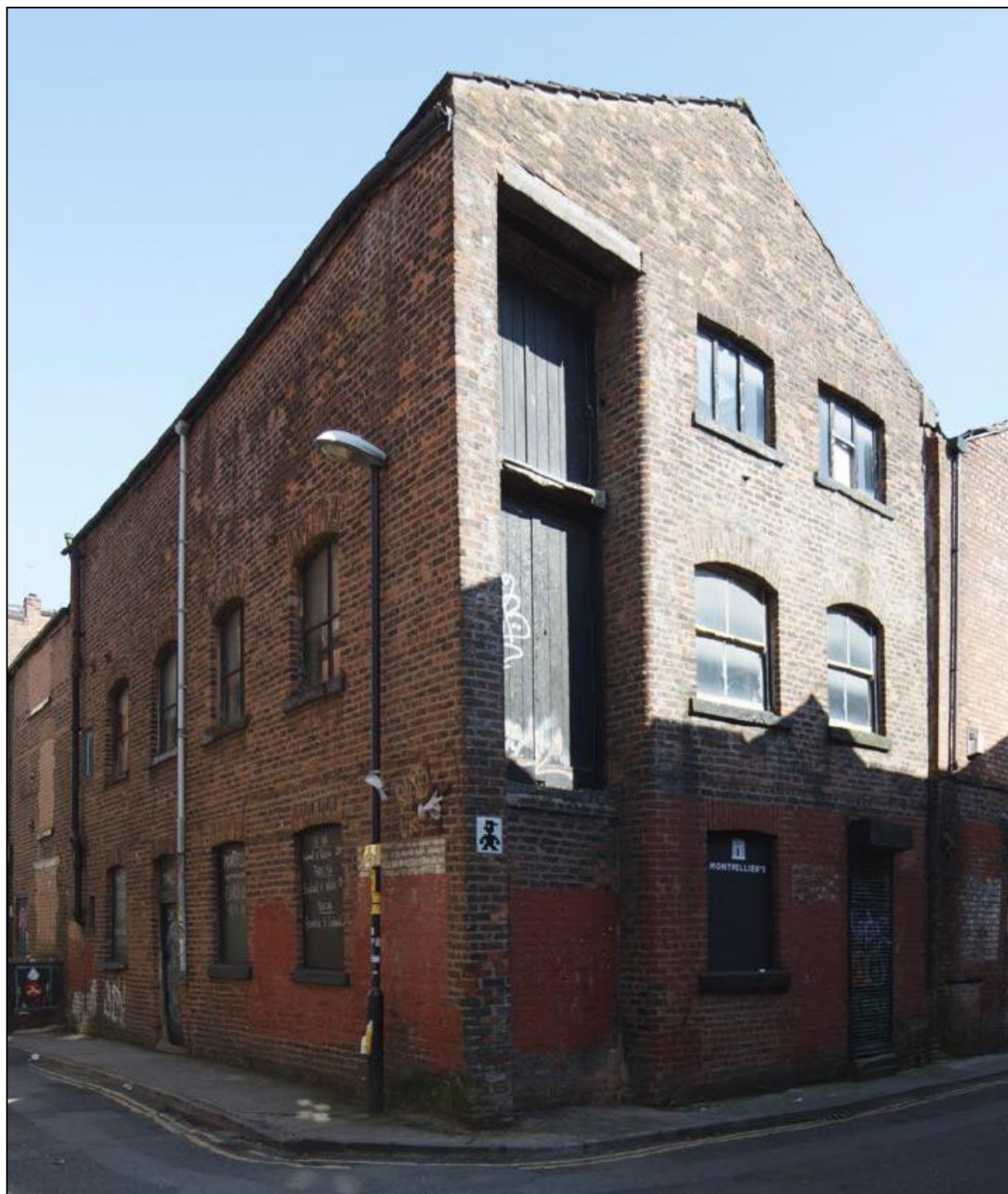
Figure 3. 7 Kelvin Street (May 2016) showing the external materials to be repaired/restored, comprising: common brick elevations, sandstone cills, timber-framed sash-windows, boarded-timber doors, slate roof, rainwater goods, fascia's and stone steps.
