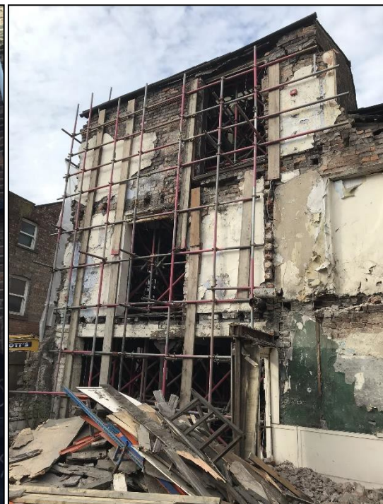
Figure 6 exposed former inner wall (2019).
