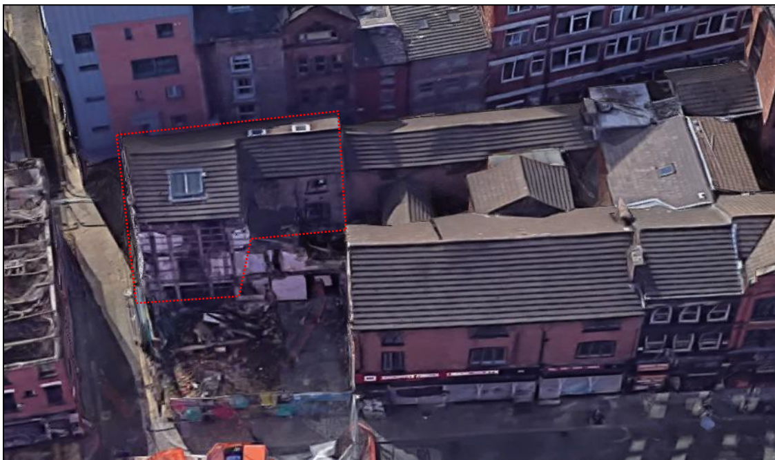
Figure 9. Aerial view of roof coverings 2018,
