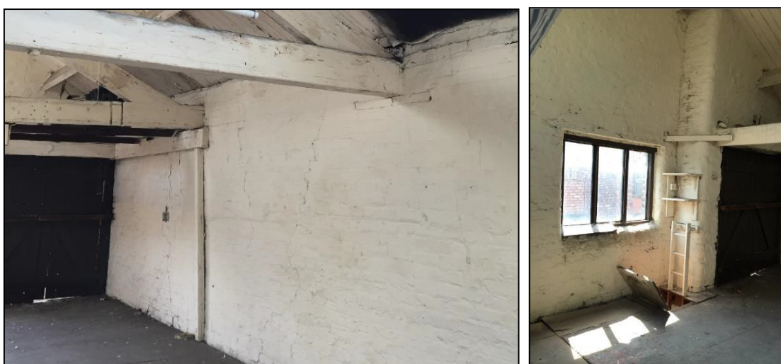
Figure 8. The lime-washed interior walls of the Back Turner Street elevation (May 2016).
