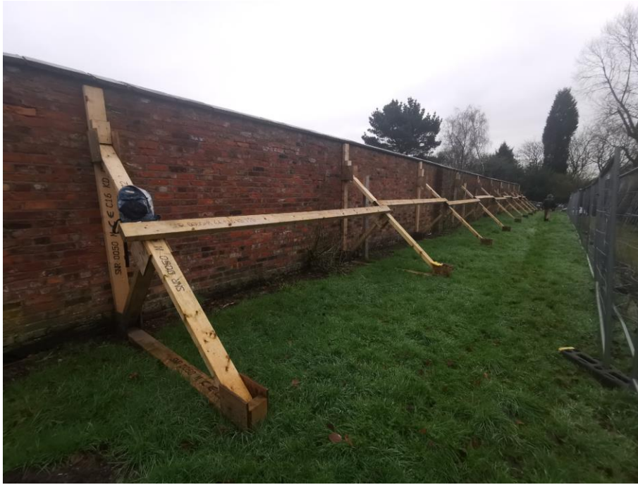
Photo 3 - Temporary Propping
