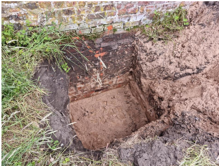
Photo 4 - Current foundation (approx. 1.2m)
