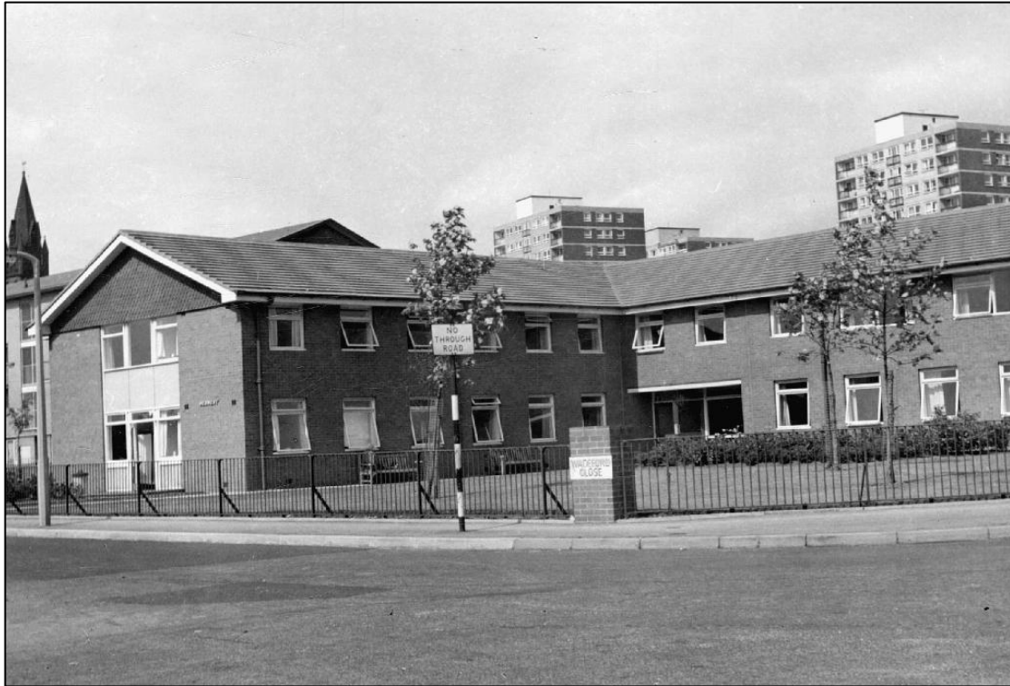
Plate 13: Redevelopment at Wadford Close taken from Rodney Street in 1967, courtesy of Manchester Local Image Collection
