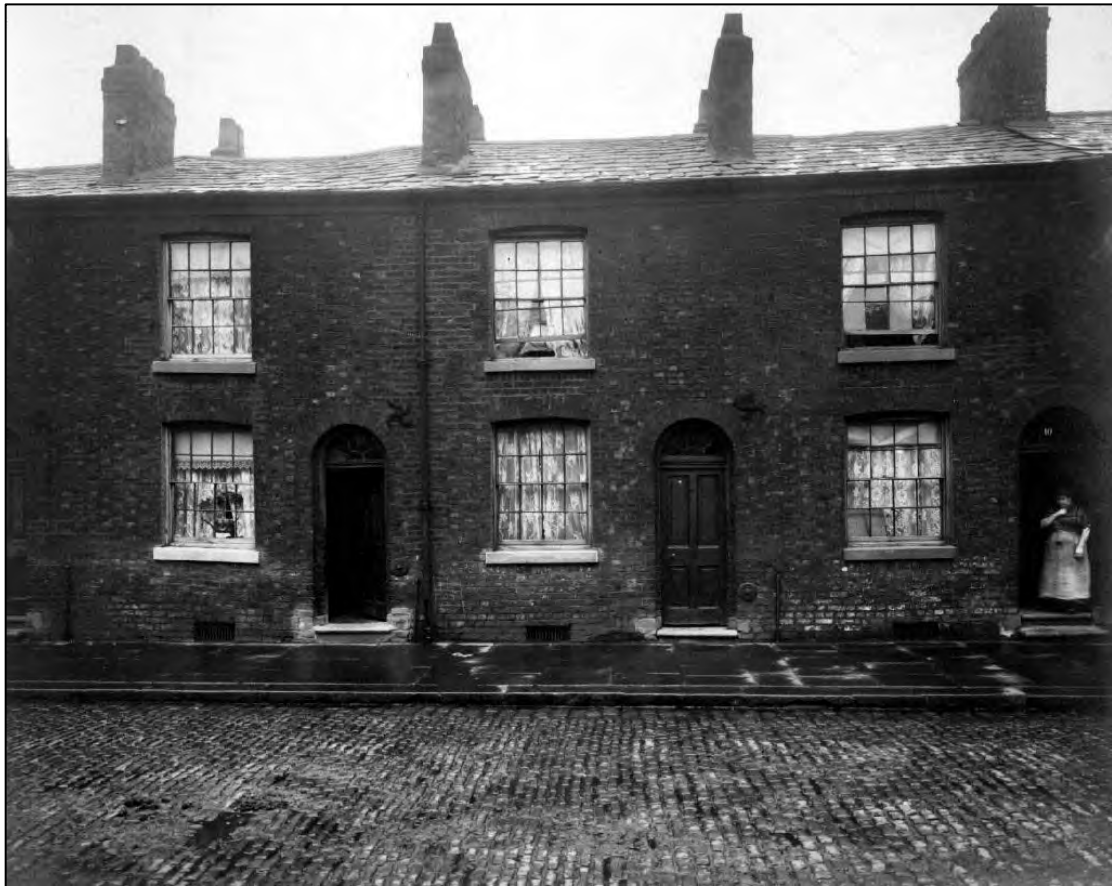
Plate 9: Elizabeth Street, Ancoats taken in 1909, courtesy of Manchester Local Image Collection
