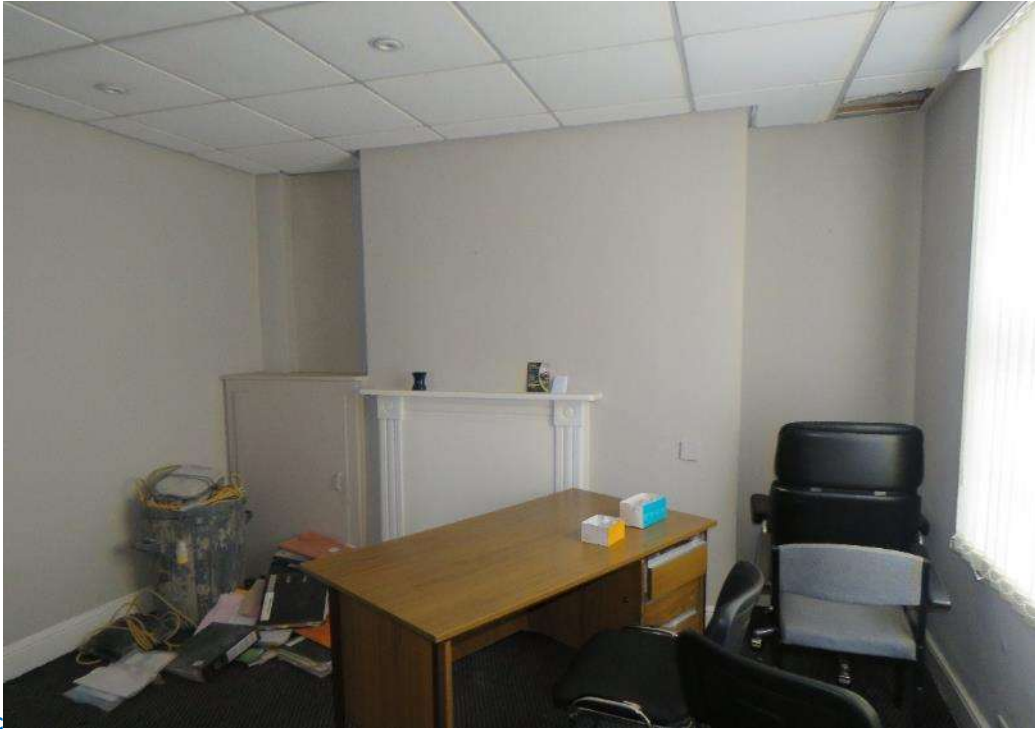
Figure 27 – The large, rear outrigger room (Room 08), showing original stone fire surround (now painted). The modern suspended ceiling covers a simple cornice.
