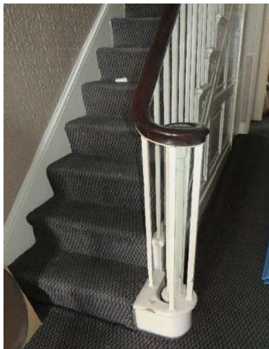
Figure 14 – The original staircase with hardwood handrail (Room 02).
