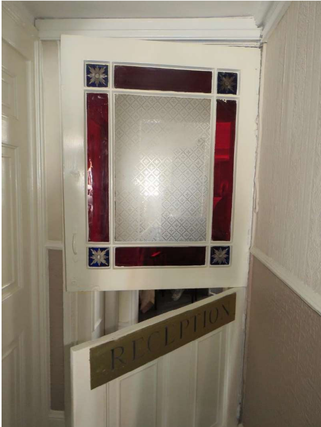
Figure 18 – A later 19 th century half-glazed door leading from the hall into the rear of the building (Room 05), featuring etched blue and red glass spandrel panels. This door has been split in half to form a reception counter.
