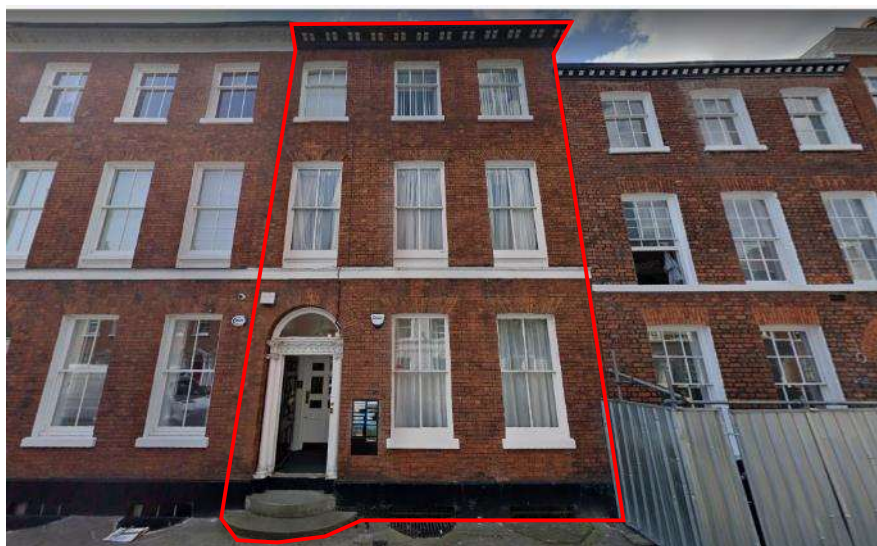
Figure 1 – The principal north front of No.17 St John Street (outlined).
