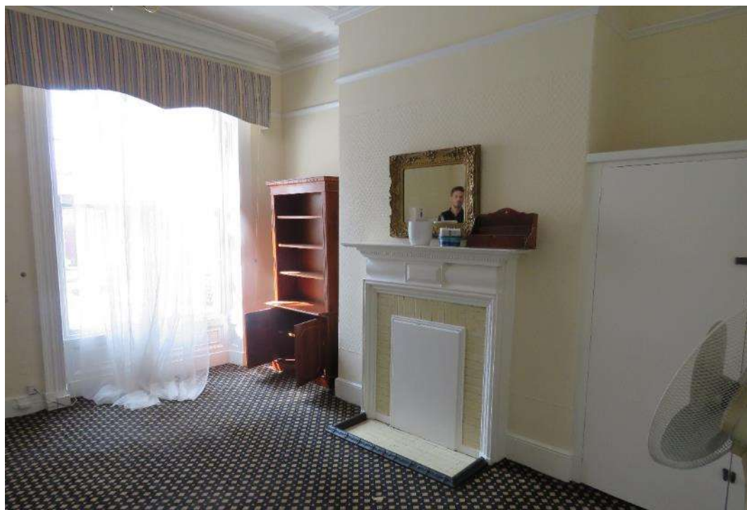
Figure 31 – Room 10 showing the original plaster cornice, simpler original skirting, and an Edwardian fire surround with fender.
