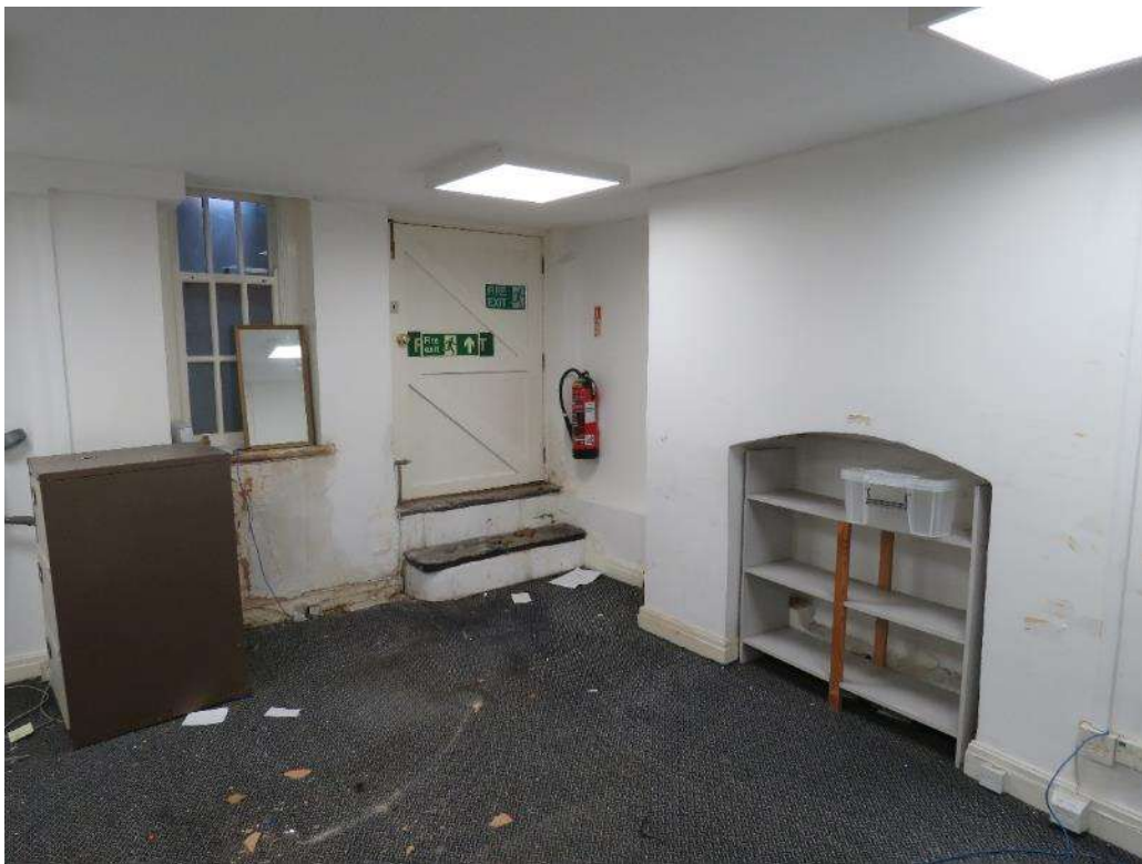
Figure 44 – The rear room (Room 20) showing the modern plastered walls, joinery, door, ceiling and sash window.
