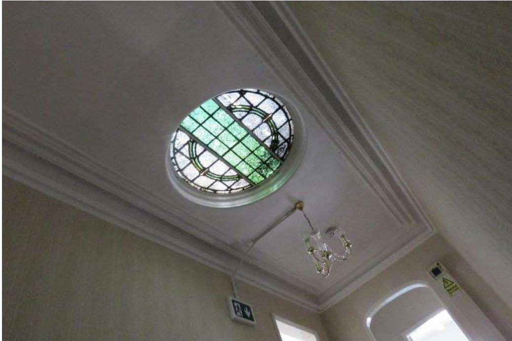
Figure 34 – The circa late-19 th century stained glass laylight to the top of the staircase (Room 11), which is fitted into the original c1820 circular opening. The same circular opening can be seen in No. 13 and No. 11 St John Street. Note the original deep plaster cornice.
