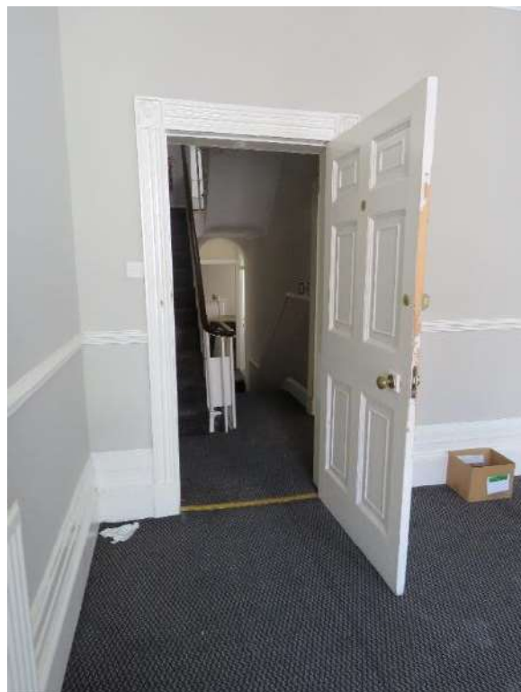
Figure 29 – The original panelled door into Room 09 (as viewed from inside Room 09). Note the original decorative brass door knobs.
