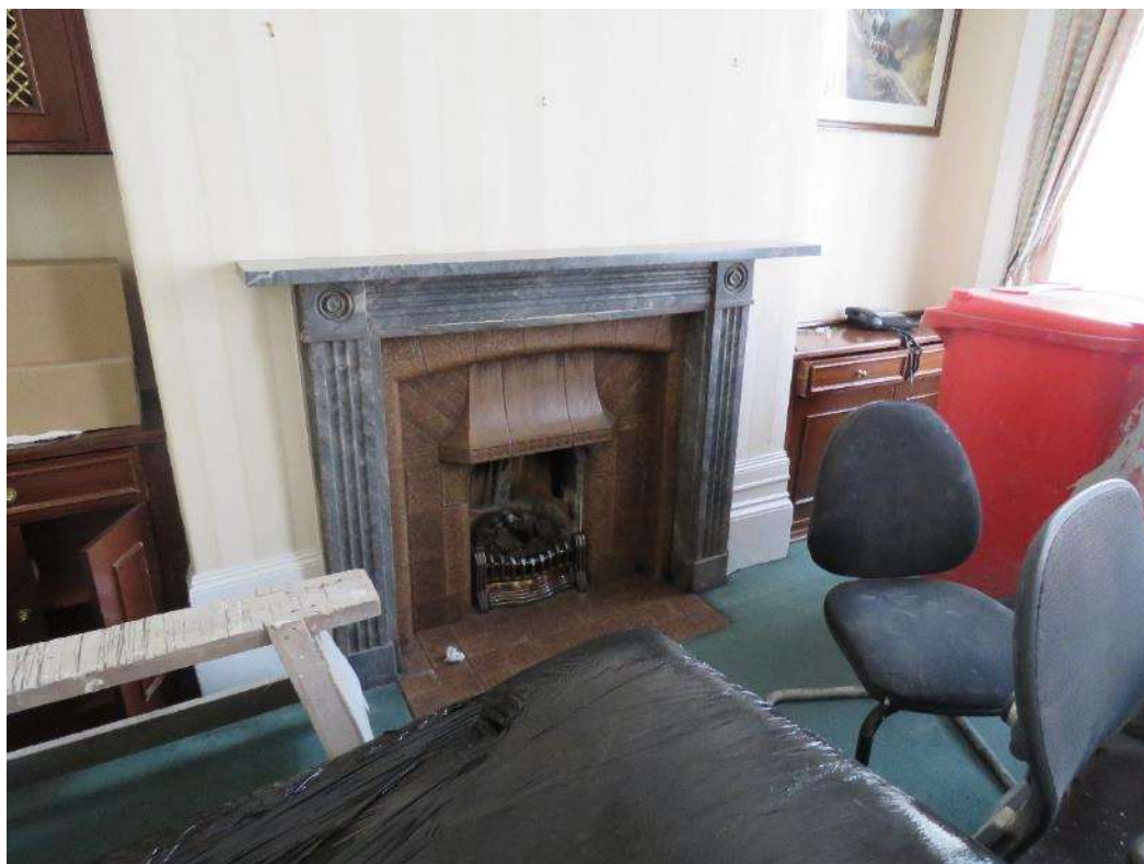
Figure 19 – The original grey/blue marble fire surround to the front room (Room 03) which contains a c1950s tiled insert and hearth .
