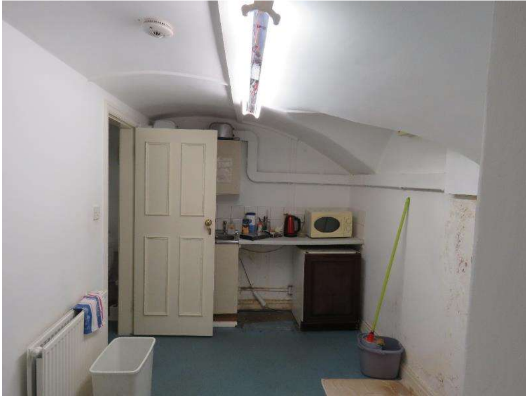
Figure 45 – Beneath the rear outrigger (Room 21), showing the original barrel-vaulted ceiling. Note the modern plastered walls, joinery and door.
