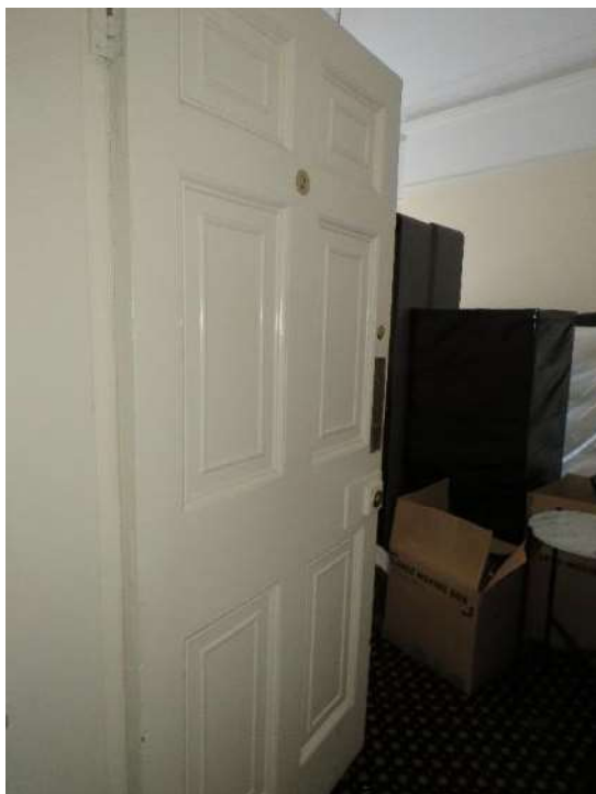
Figure 22 – Looking into the rear reception room (Room 04), showing the original panelled door.
