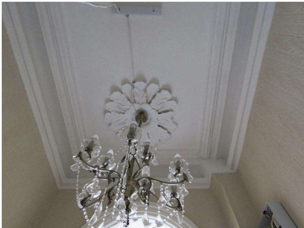
Figure 16 – The original decorative plaster ceiling rose and cornice to the entrance hall.
