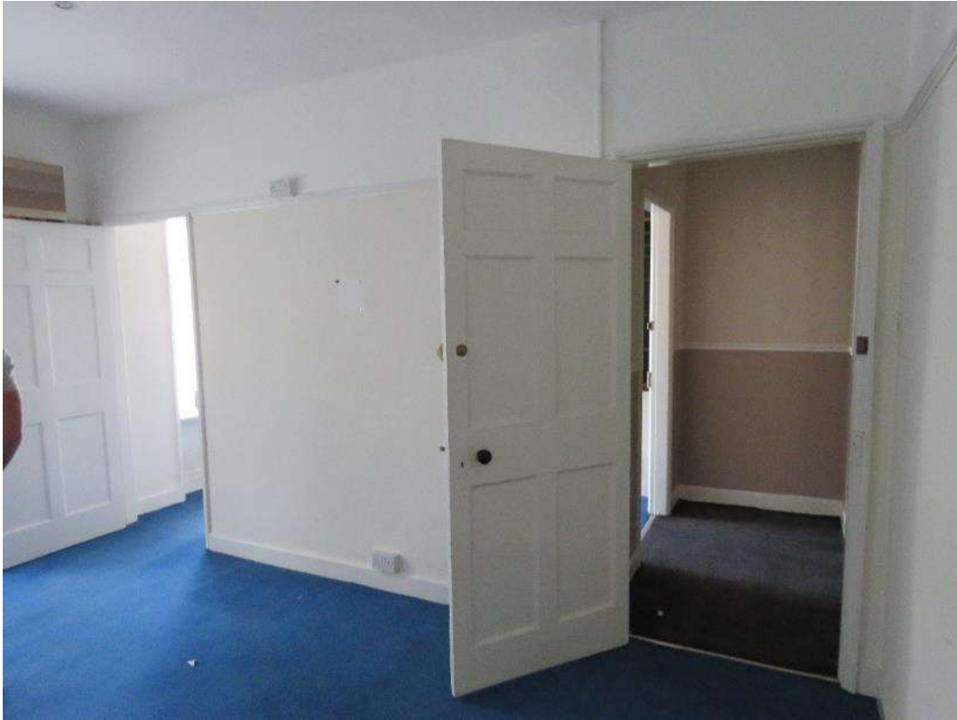
Figure 36 – Looking east across Room 12 showing the much simpler original six-panelled door without the use of inner beading.
