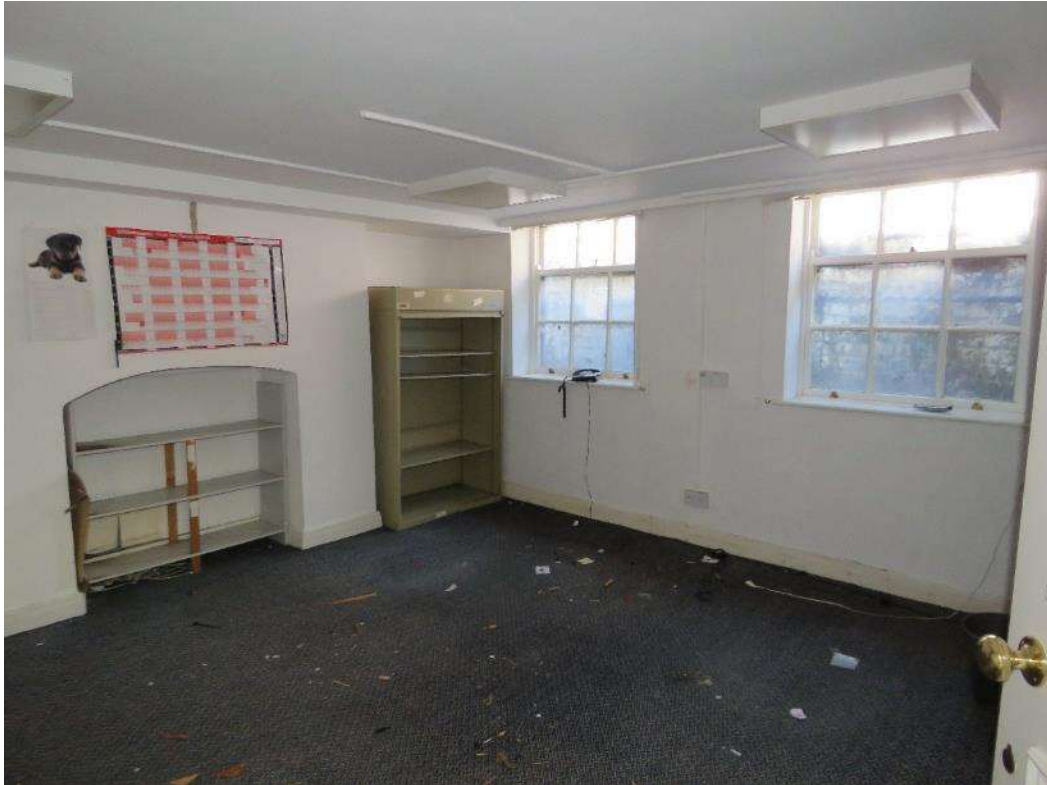
Figure 43 – The front room (Room 19), showing the modern plastered walls, joinery, ceiling and sash windows.
