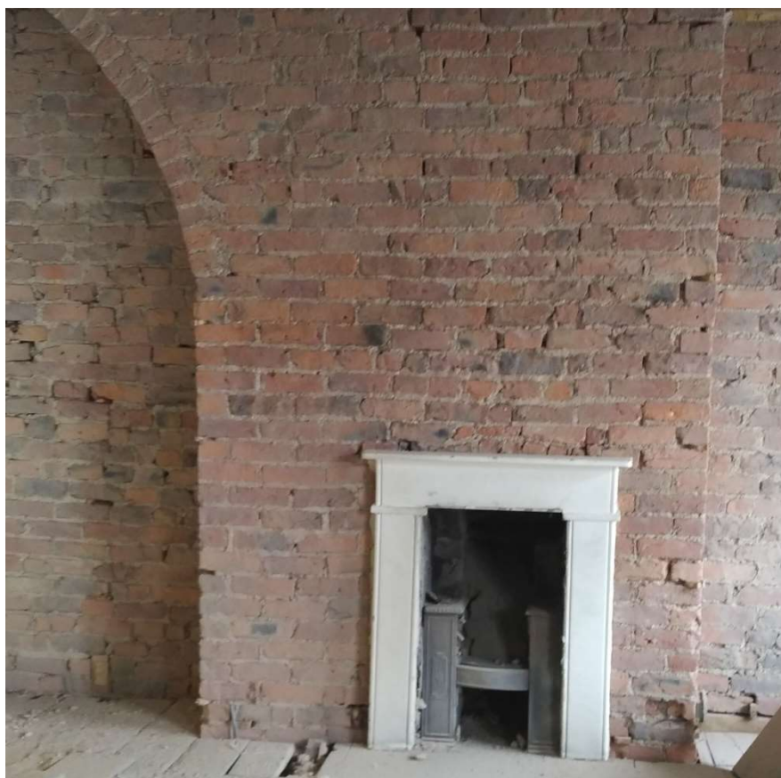
Figure 39 a – Newly uncovered cast-iron hob grate; arched chimney breast; and exposed brickwork
