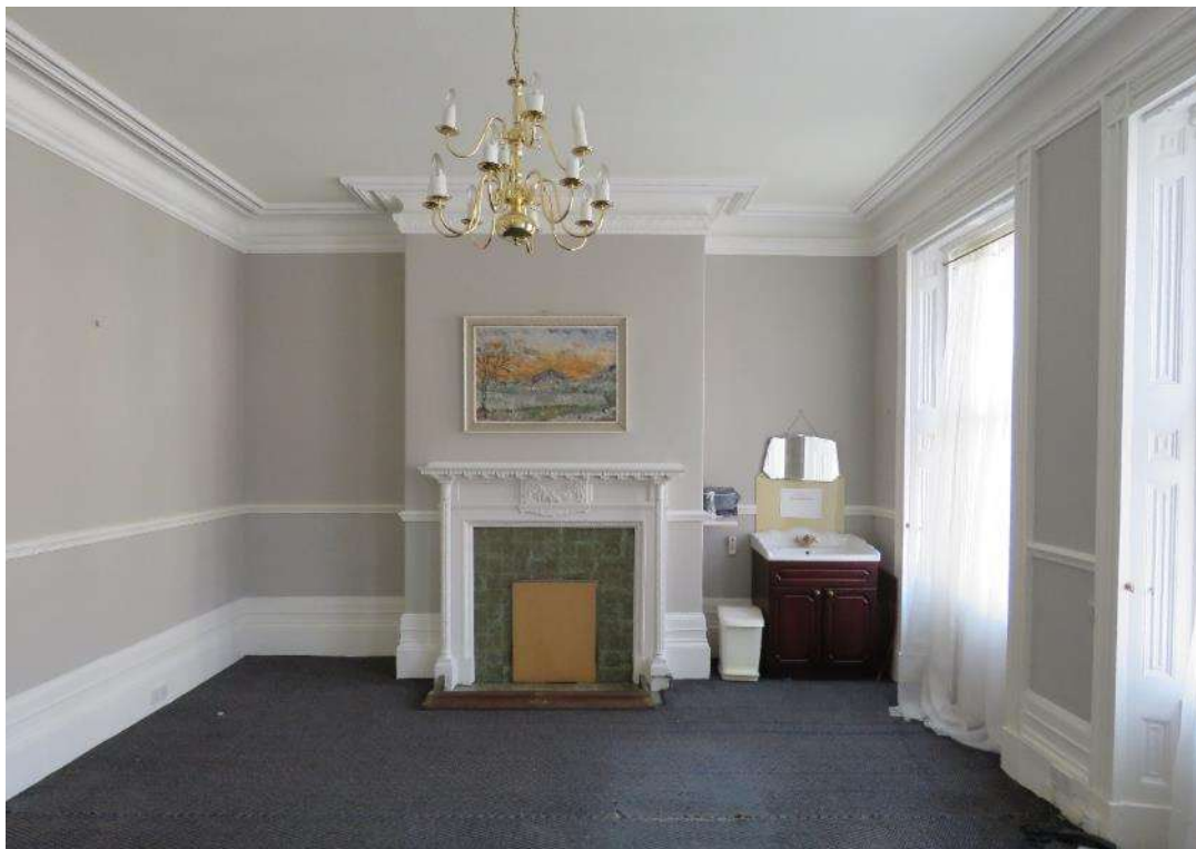
Figure 28 – The former principal bedroom (Room 09) showing the very deep moulded skirting boards, dado rail, deep plaster cornice and a later-19 th century timber fire surround (with 20 th century tiled insert) and period brass hearth fender.
