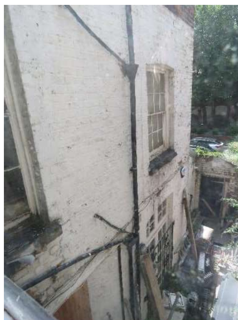
Figure 47 – The rear outrigger as seen from Room 10, showing the original multi-pane sash window to Room 08 (with Edwardian patterned glass), and modern windows to the Ground Floor level.
