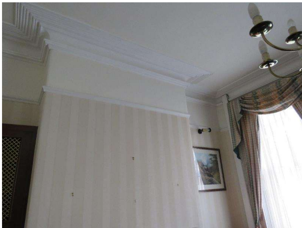
Figure 20 – The deep original plaster cornice to the front room (Room 03).
