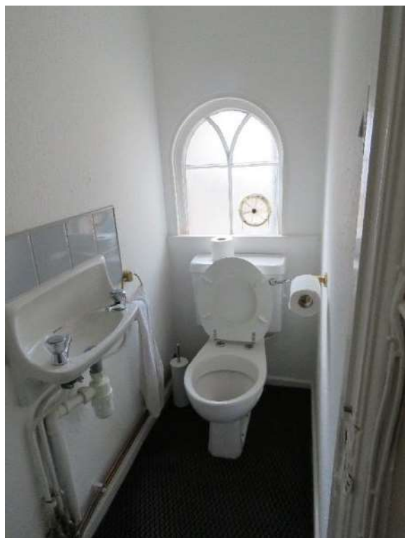
Figure 39 – The modern WC (Room 16), which appears to be located in what was originally a double-height servant's staircase, linking the Second Floor with the First Floor below.
