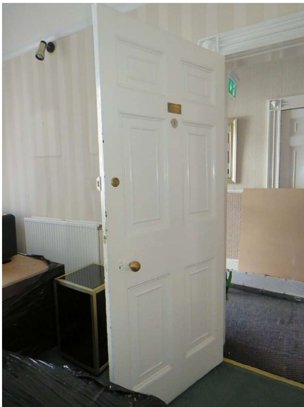
Figure 21 – The original panelled door into Room 03, showing an original/early brass beehive door knob.
