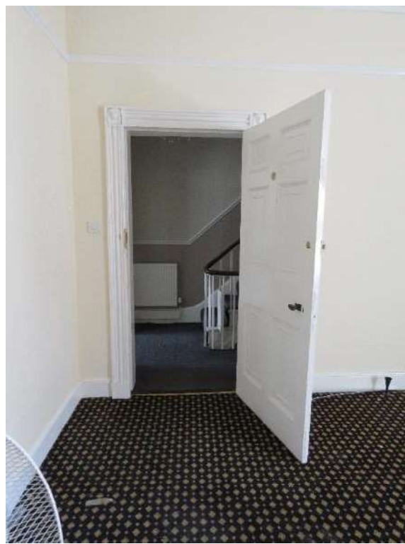
Figure 30 – The original panelled door into Room 10, as viewed from inside Room 10) with Edwardian brass doorknobs.
