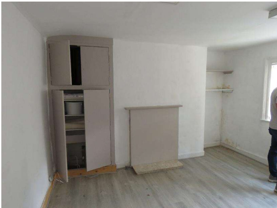
Figure 38 – Room 15, again illustrating the simpler design of these Second Floor rooms. The original fire surround may be concealing a surviving cast iron fire insert behind modern boarding.
