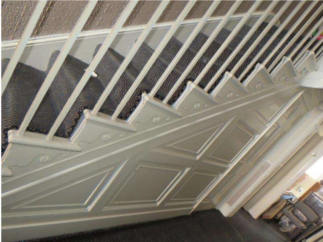
Figure 17 – The panelled staircase showing the original basement door (right) which has since been sealed shut.
