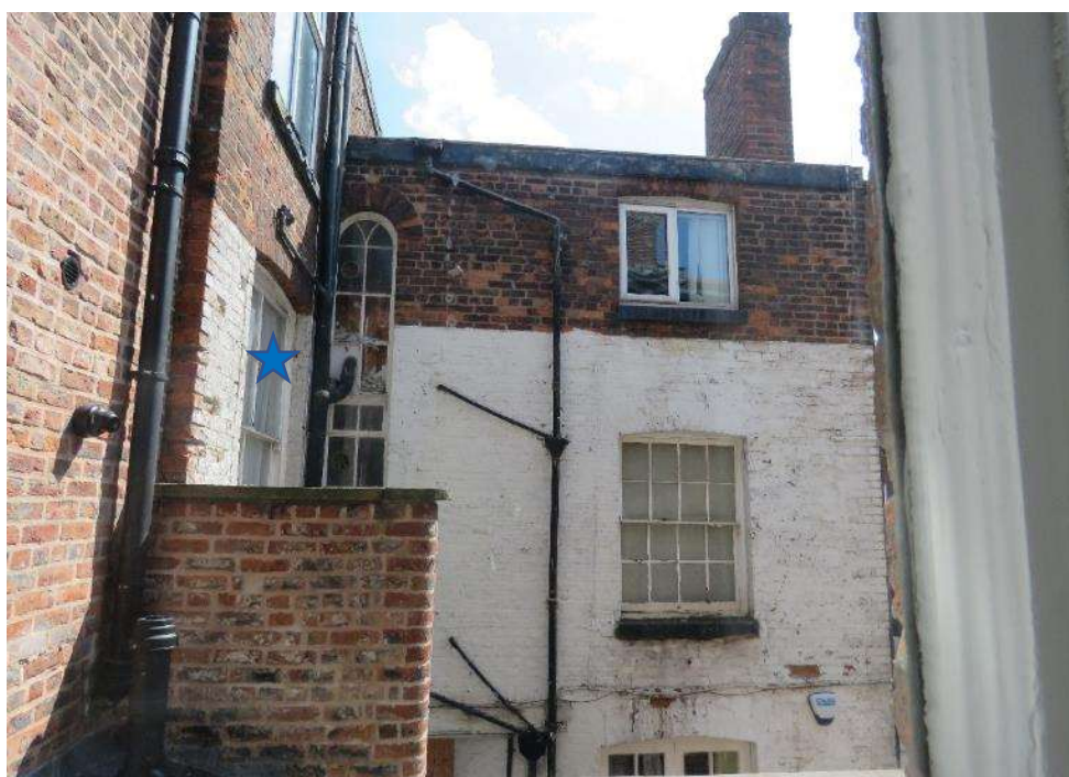
Figure 48 – Looking east towards the rear outrigger of No. 17 (as seen from No. 19 St John Street) showing the modern painted brickwork, modern UPVC Second Floor windows, later-19 th century window (marked by blue star) and narrow, double-height sash window (left) which retains its original upper half (Rooms 07 & 16).
