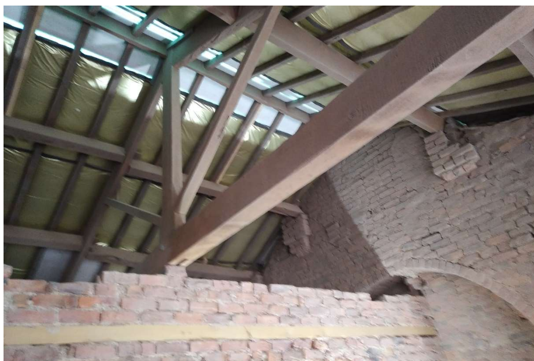
Figure 39 b – King-post truss revealed
