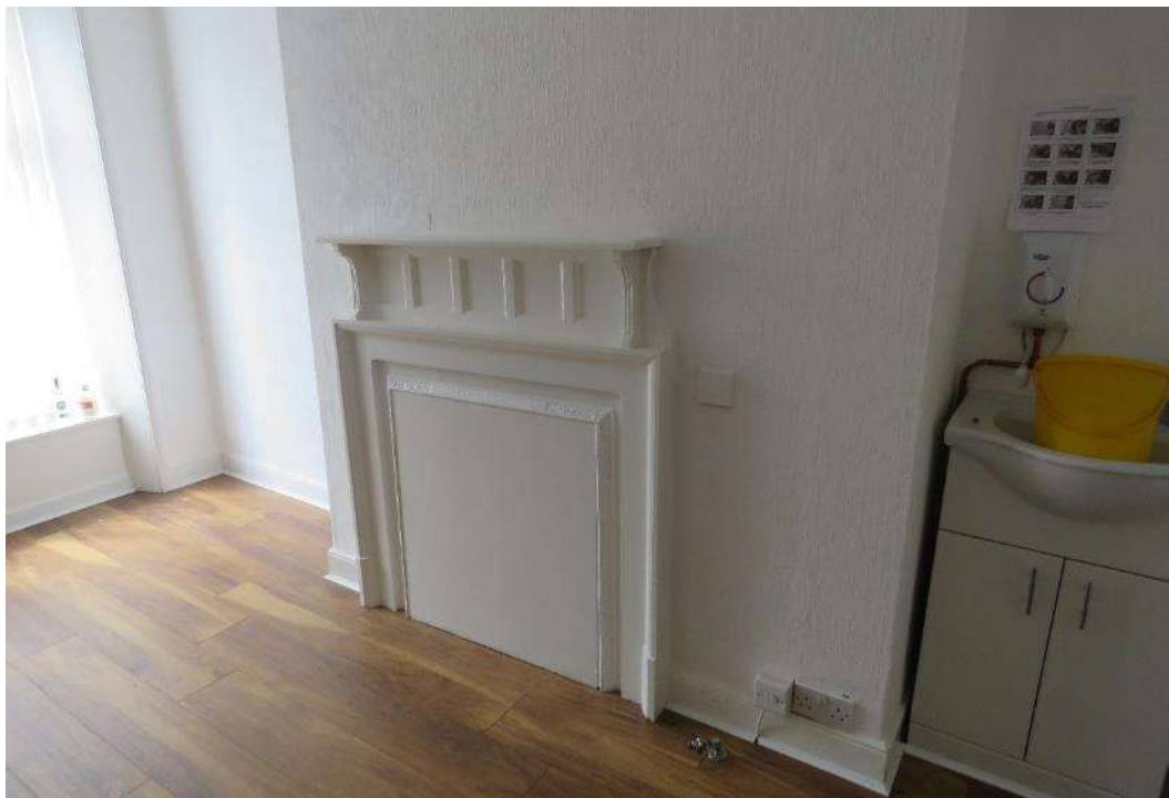
Figure 37 – A late-19 th century timber fire surround to Room 14 (which may be concealing a surviving cast iron fire insert behind modern boarding).
