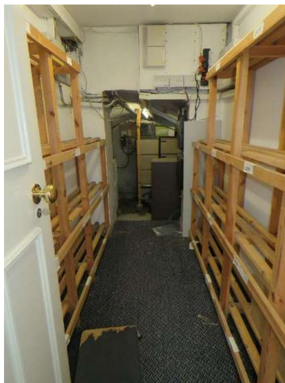
Figure 42 – Looking towards the original coal store beneath the vestibule (Room 18). Note the modern door and plasterwork.
