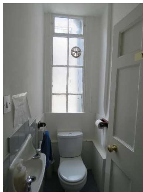
Figure 26 – The First Floor WC (Room 07), housed in what appears to have originally been the bottom of a two-storey servant's staircase leading to the Second Floor. (See Figure 48)
