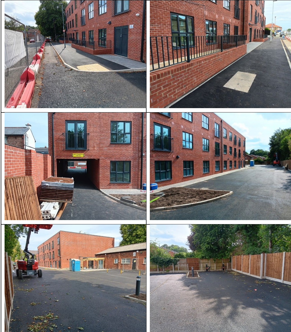
Photographs 1-6: Selected photographs of completed site.
