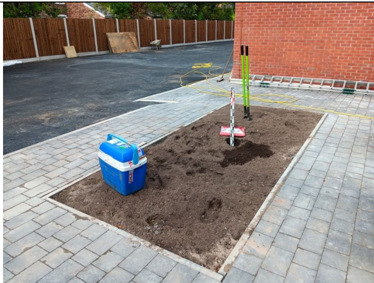
Photograph 1: View of Pit 4 location.
