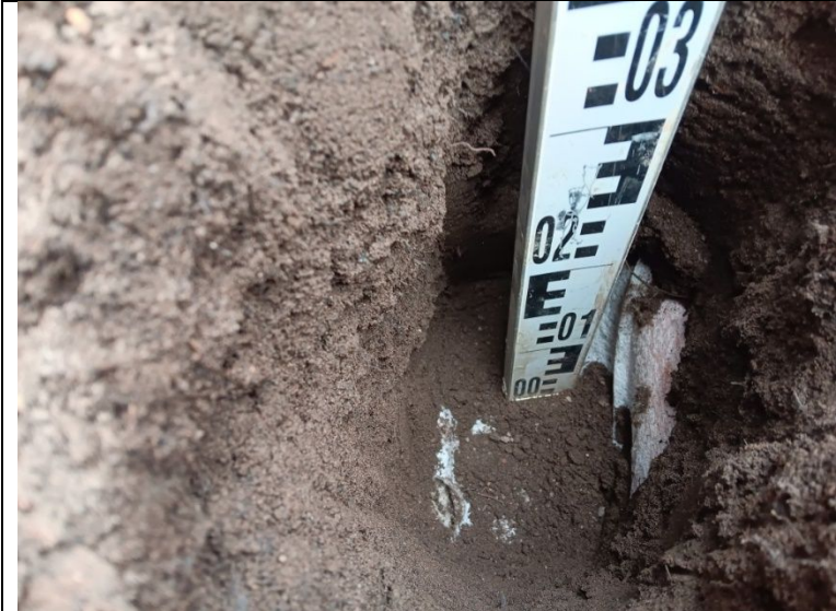
Photograph 2: View of capping layer excavation in Pit 2. Geotextile membrane present at base.
