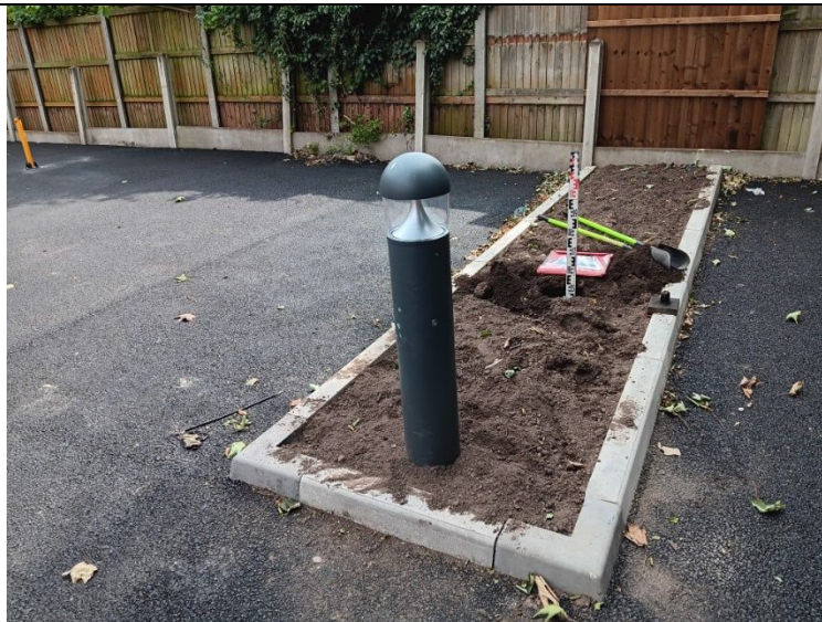
Photograph 1: View of Pit 5 location.
