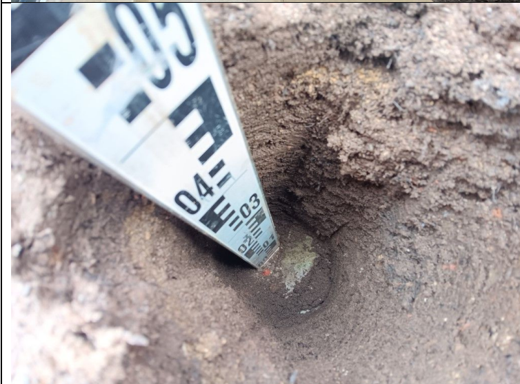
Photograph 2: View of capping layer excavation in Pit 1. Geotextile membrane present at base.
