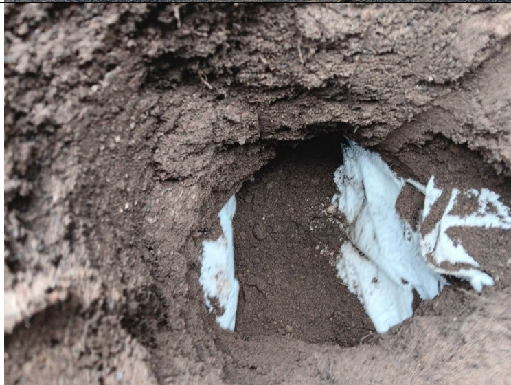
Photograph 2: View of capping layer excavation in Pit 5. Geotextile membrane present at base.
