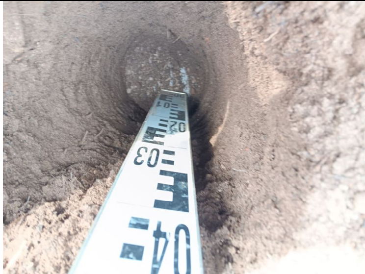
Photograph 2: View of capping layer excavation in Pit 3. Geotextile membrane present at base.
