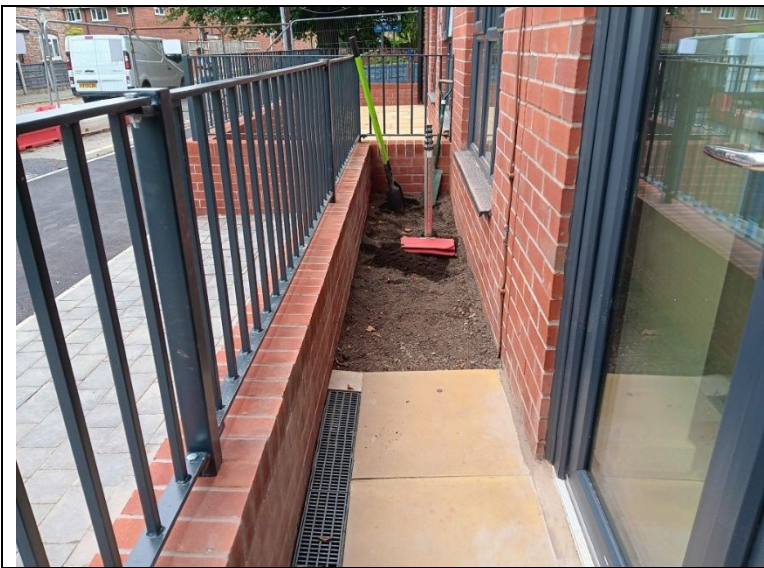
Photograph 1: View of Pit 2 location.
