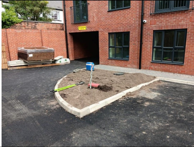
Photograph 1: View of Pit 3 location.
