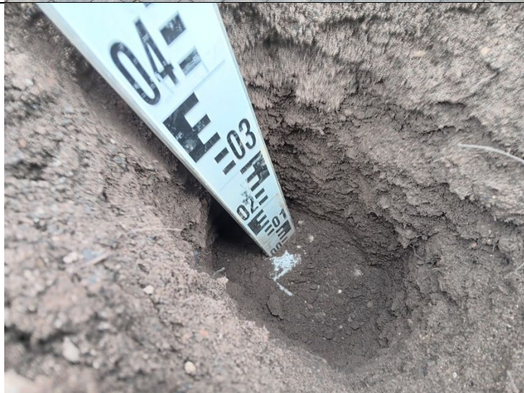
Photograph 2: View of capping layer excavation in Pit 4. Geotextile membrane present at base.
