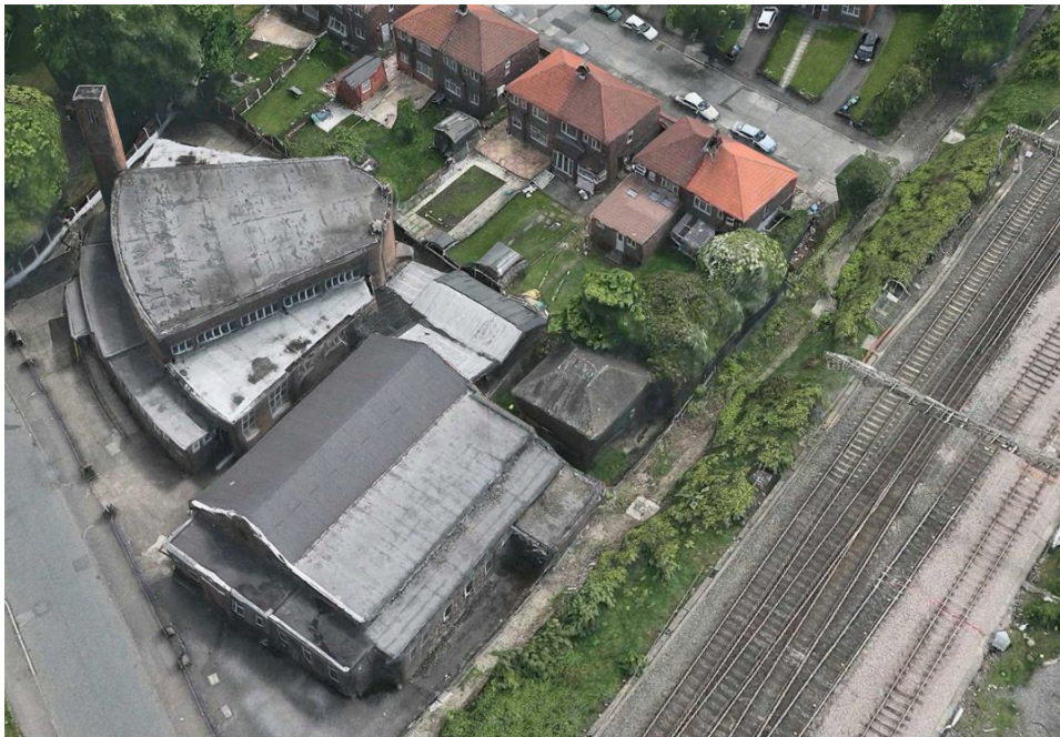
Figure 2: 3D aerial photograph indicating nearest receptors to Authentic City Church
