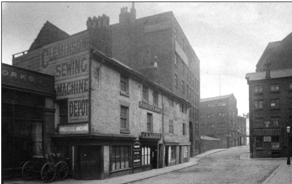
Plate 12: View of Irk Mills opposite warehouse at the junction of the Hanover Street, also shows the adjacent weavers' cottages, three of which are located within the Site, taken in 1900, courtesy of Manchester Local Image Collection
