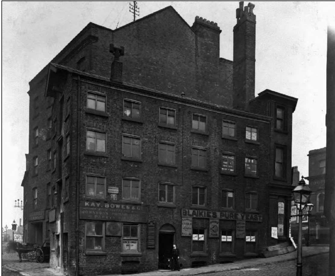
Plate 11: Warehouse at the junction of Hanover Street and large remodelled building at Long Millgate taken in 1900, courtesy of Manchester Local Image Collection
