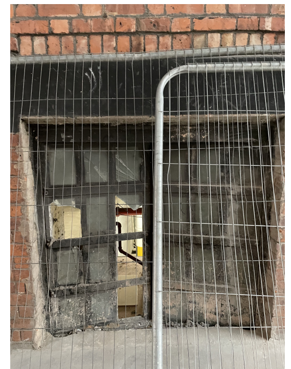
Photograph of existing opening 10/03/22
