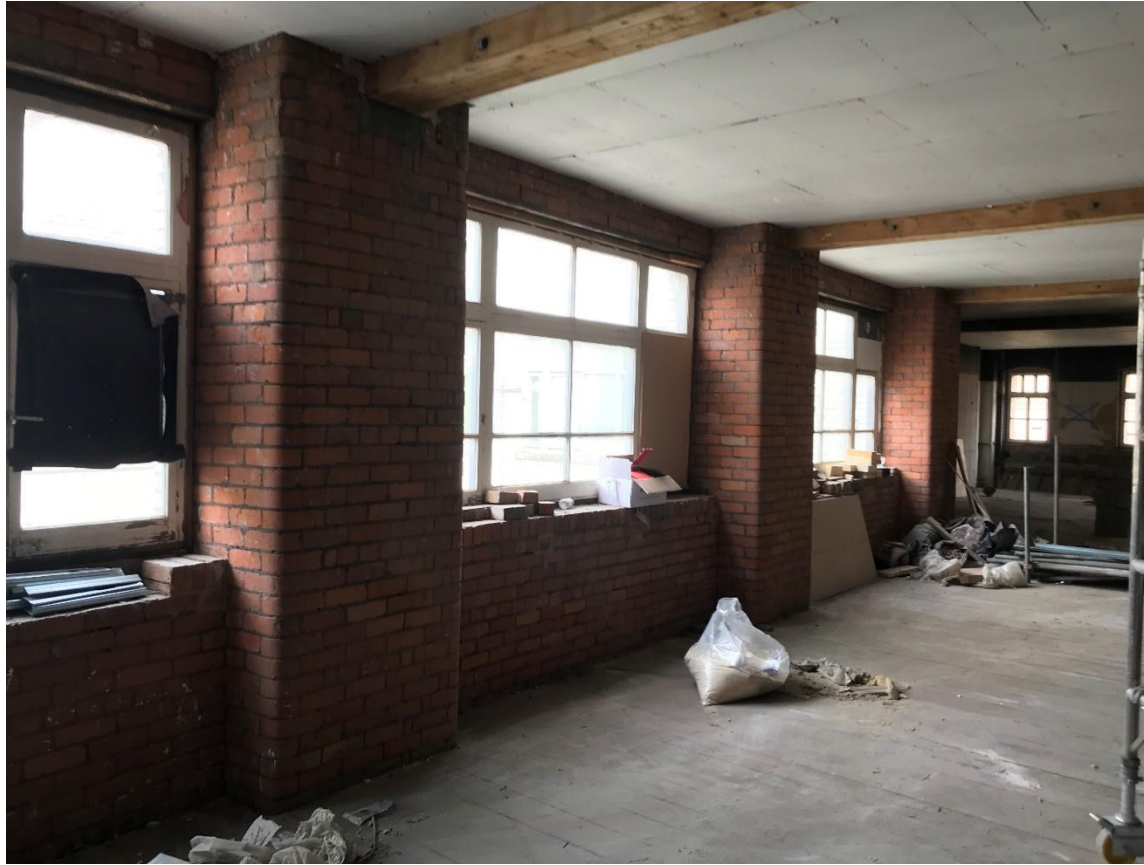
Figure 25: Brick Piers 1 (Credit CubicWorks Ltd. 2022)
