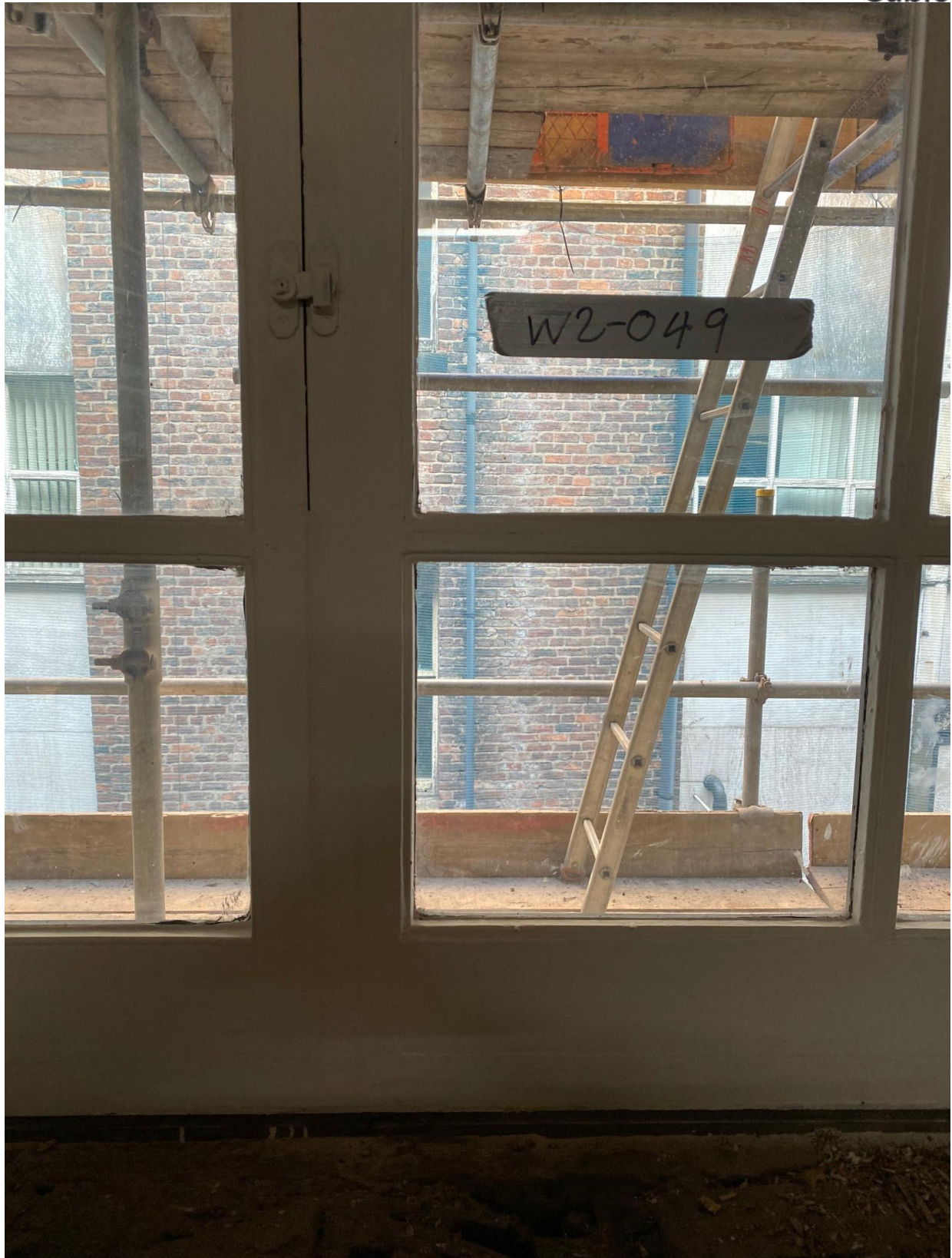
Figure 7: W2-049 Window painted after repairs (Credit CubicWorks Ltd.2022)
