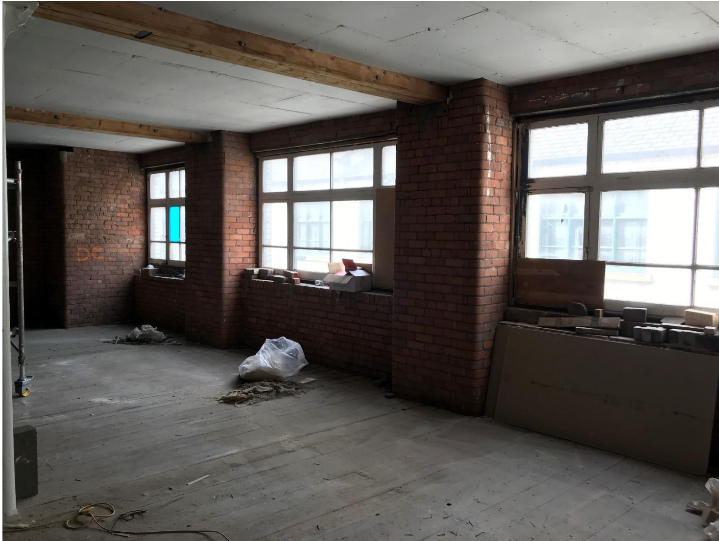
Figure 27: Brick Piers 3 (Credit CubicWorks Ltd.2022)
