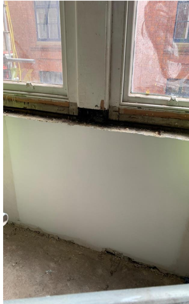
Figure 22 : Paint to Lime plaster wall – Level 5 - GRAPHENSTONE GLACIER GRAFCLEAN INT (Credit CubicWorks Ltd.2022)
