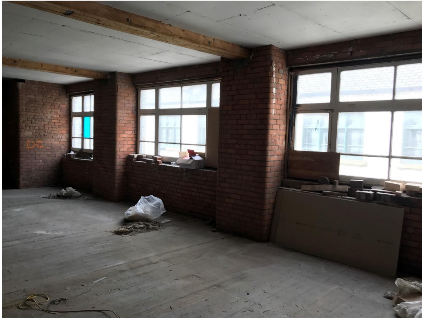
Figure 26: Brick Piers 2 (Credit CubicWorks Ltd.2022)
