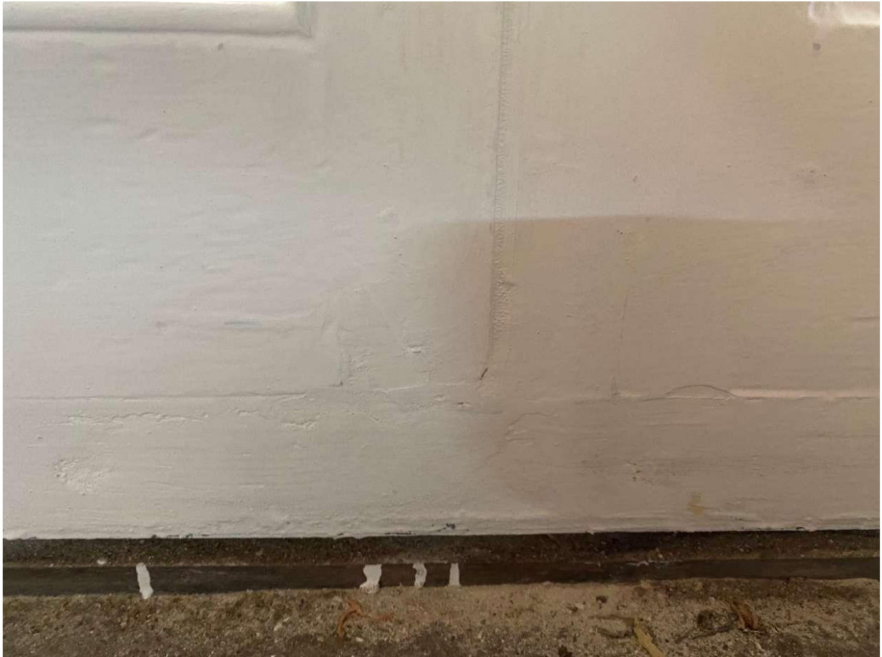
Figure 5: W2-049 Decorative finish (Credit CubicWorks Ltd.2022)
