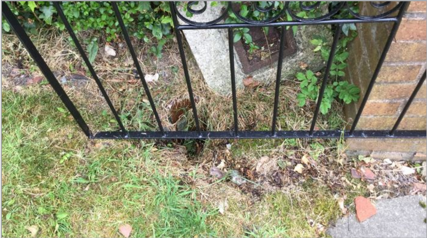
Exposed gulley in front garden
