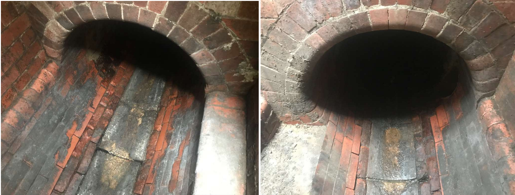
Images 1 & 2 showing the construction of the Collyhurst 'V' Sewer at the entry manhole closest to site
