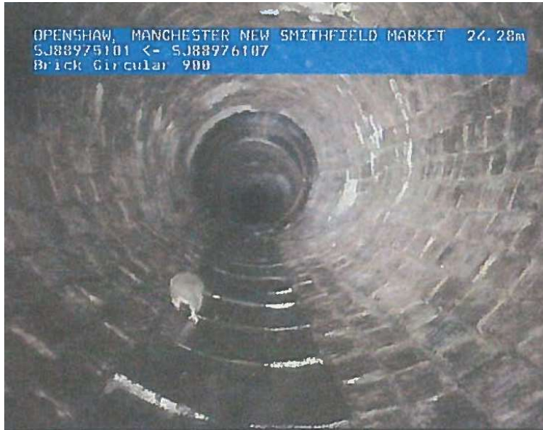
Image 3 & 4 showing the condition of the 900mm diameter Collyhurst 'V' sewer
