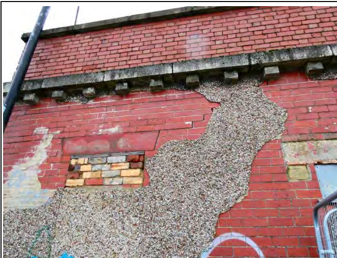
Decorative Stone Cornice and Parapet Rough Cast Render - Infilled Openings
