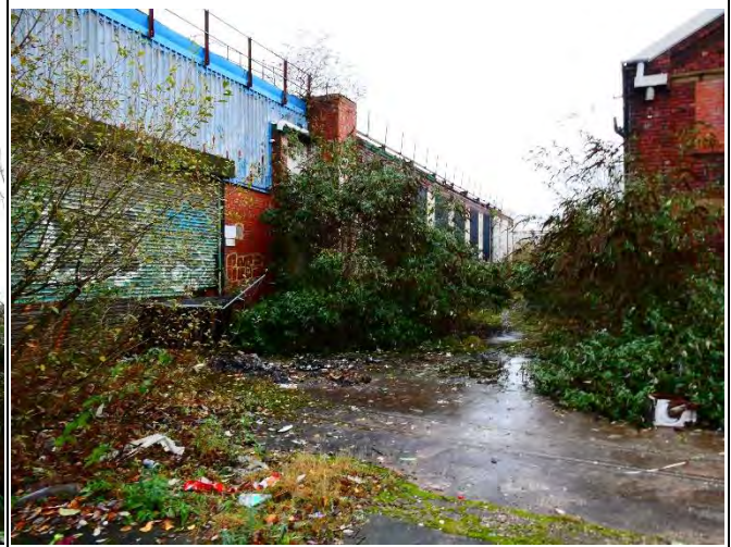
East Elevation of Area 13
