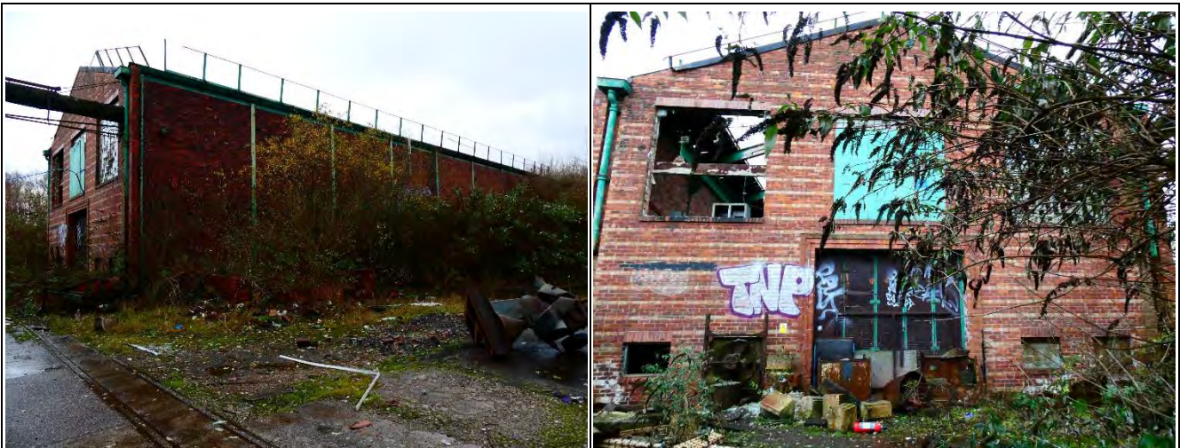
North and West Elevation of Area 16
