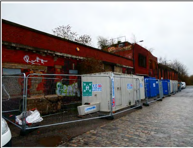
West Elevation of Area 4 Along Crabtree Lane
