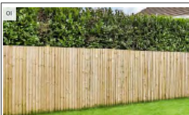
Proposed 1800mm Close Boarded Timber Fence
