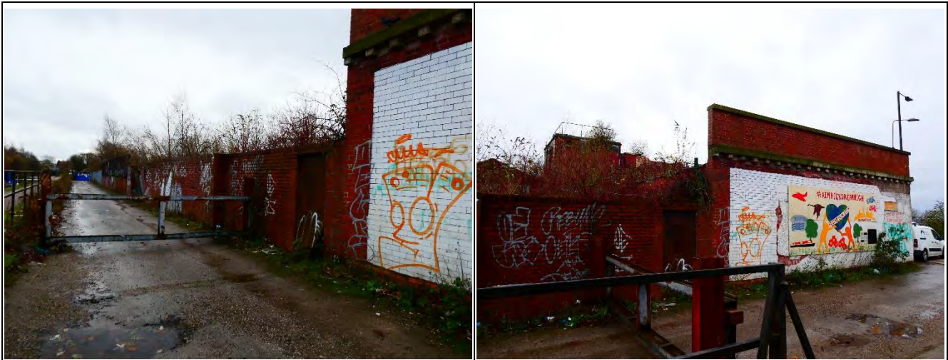
North Boundary to the Proposal Site Looking East (Along the Towpath of Ashton Canal)
