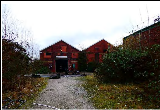
South Elevation of Area 8
