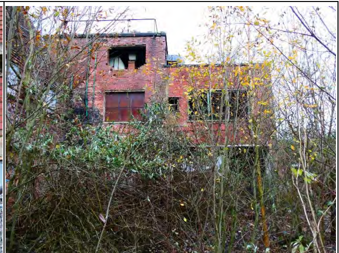
East Elevation of Offices (Area 4)
