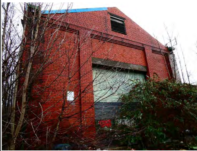
South Elevation of Area 13
