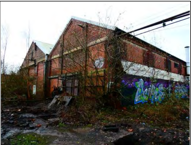
North Elevation of Area 8
