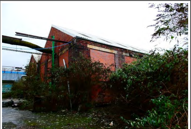
South and East Elevations of Area 8
