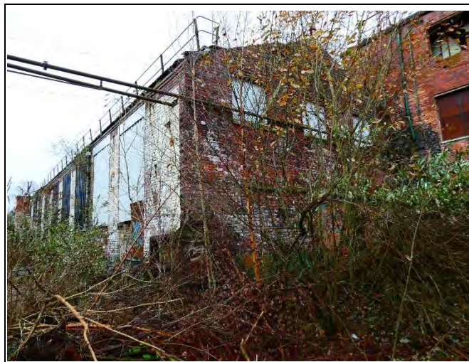
North Elevation of Area 13
