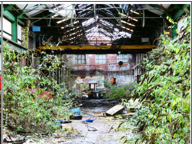
Remnants of an Overhead Crane
