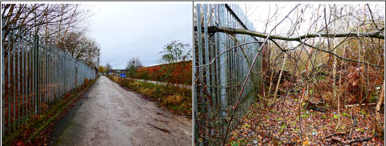
North Boundary Metal Security Fencing Looking West Along the Towpath of the Ashton Canal
