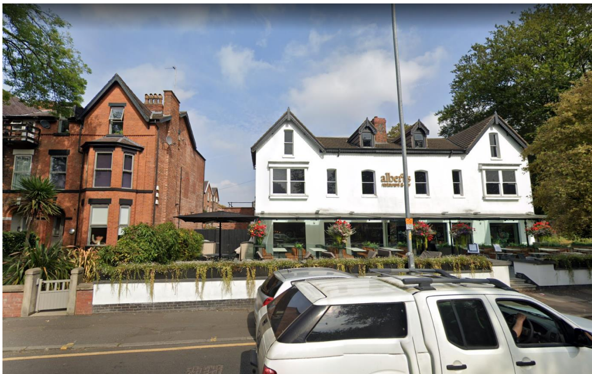
Figure 4. Image of the façade of the building and neighbouring house taken from Barlow Moor Road to the south. The existing single storey extension can be seen between the two where the proposed upper floor extension is to be situated. This image is intended to demonstrate the impact of the proposal on the architectural interest attributed to the building and its neighbour and their setting.
