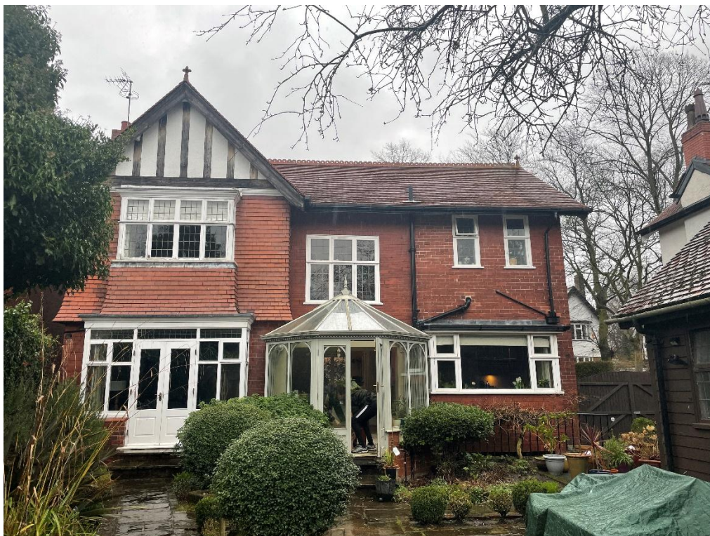
Rear of 4 Pine Road – conservatory and kitchen bay to be demolished
