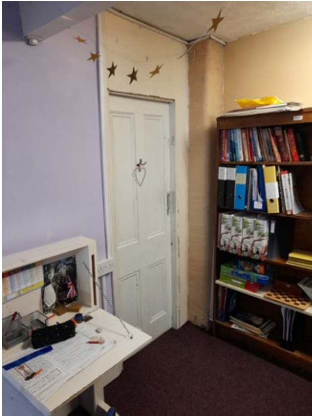
3.2.4.47 Fourth Floor, Fo1 (Install)
