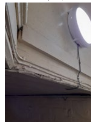
Third Floor, Stair Adj to T19
