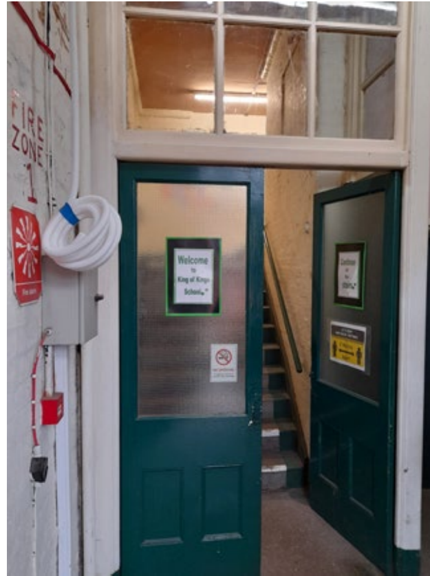
3.2.1.2 Ground Floor, G13 (Install)
