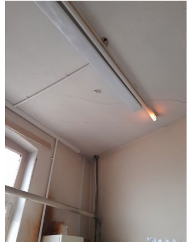
3.2.4.32 Third Floor, T16 (Install)
