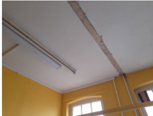
3.2.4.31 Third Floor, T15 (Install)
