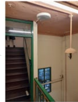
Stair between second and third floor
