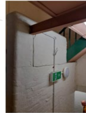
Stair between first and second floor
