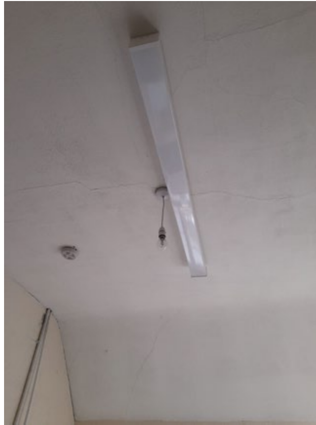
3.2.4.4 Third Floor, T1 (Install)
