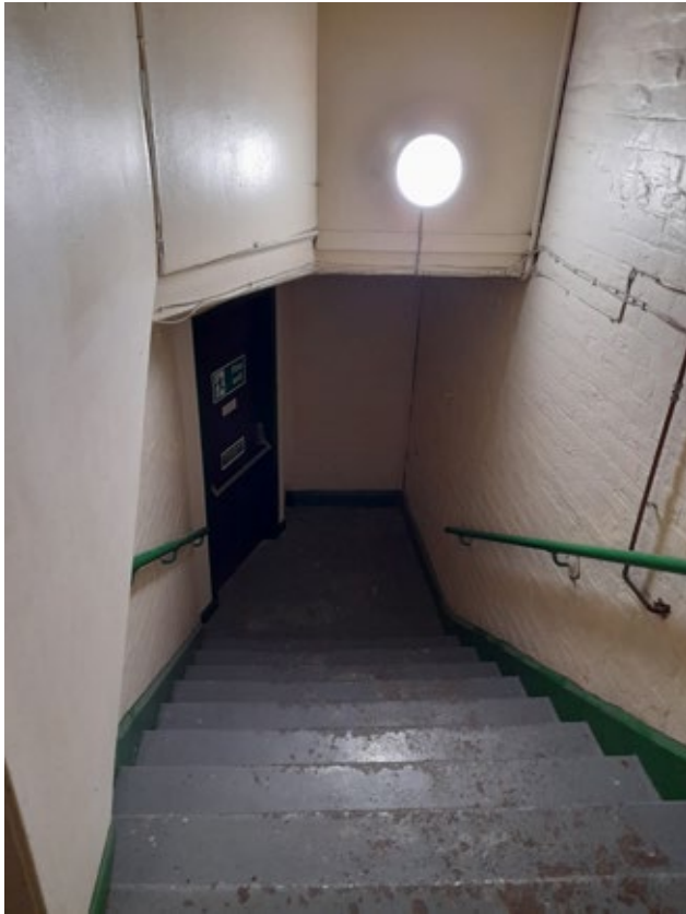
3.2.4.39 Third Floor, Stair Adj to T19 (Insall)
