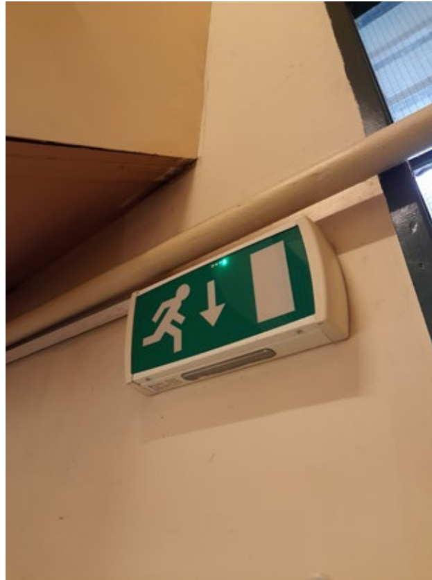
3.2.3.2 Stair S16 (Install)
