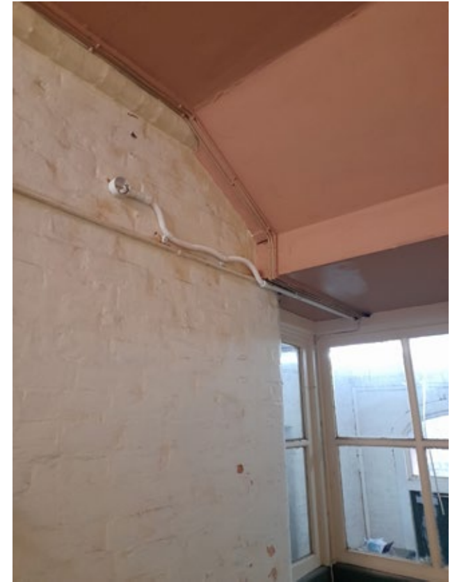
3.2.2.3 First Floor, Stair, F19 (Install)
