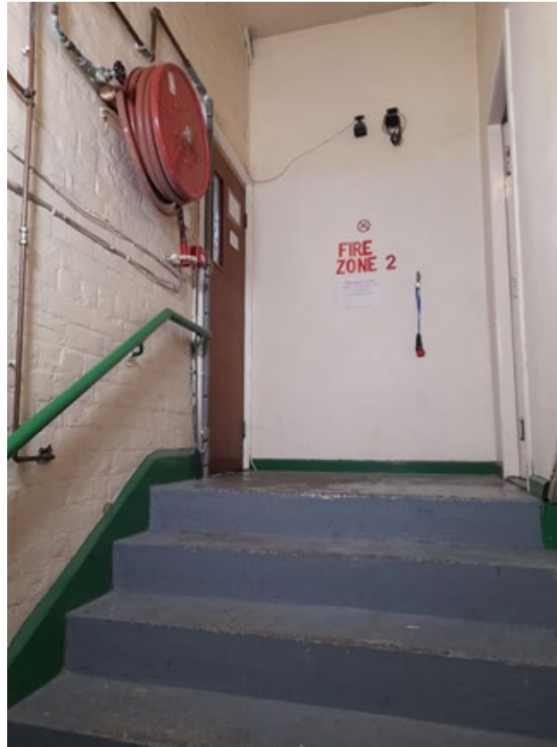
3.2.4.40 Third Floor, Stair Adj to T19 (Insall)
