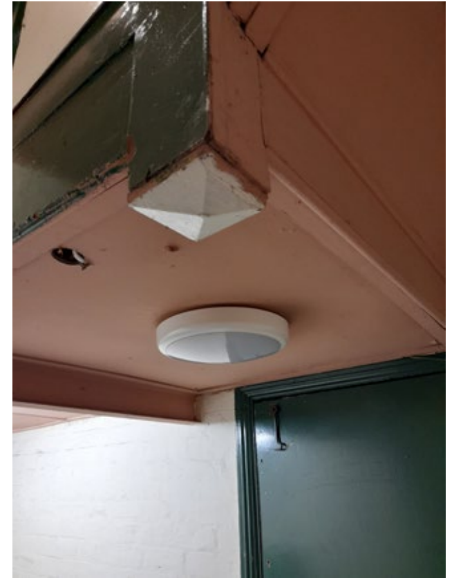
3.2.3.3 Stair S16 (Install)
