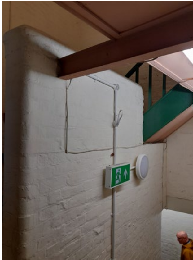
3.2.3.5 Stair S16 (Install)
