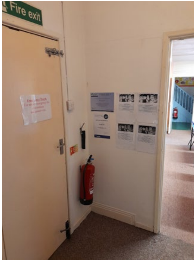
3.2.4.6 Third Floor, T3 (Install)
