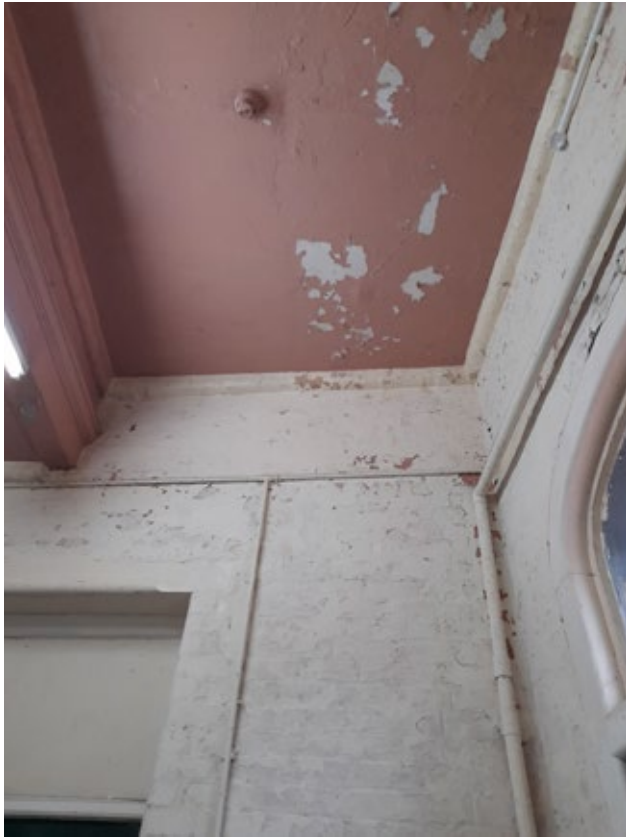
3.2.1.1 Ground Floor, G13 (Install)
