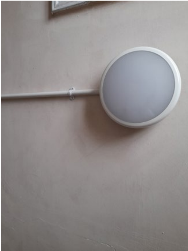
3.2.3.4 Second Floor, Stair S4 (Install)
