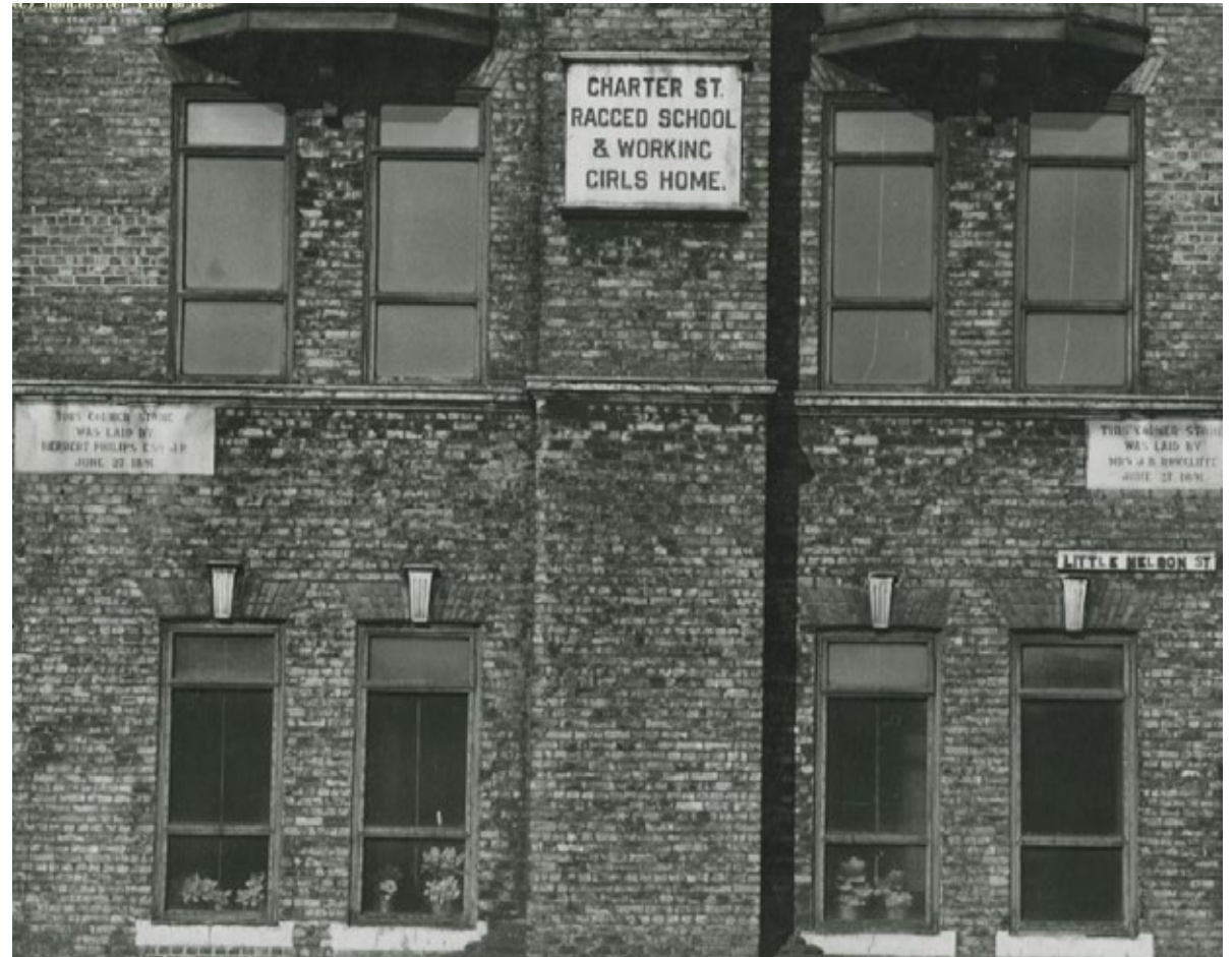
2.34 Aspin Lane (south) elevation, 1958 (L. Kaye, Manchester Archives)
