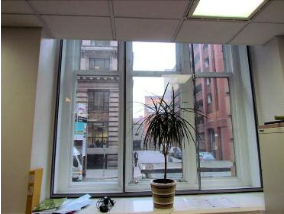
Figure 5: Secondary Glazing, Office
