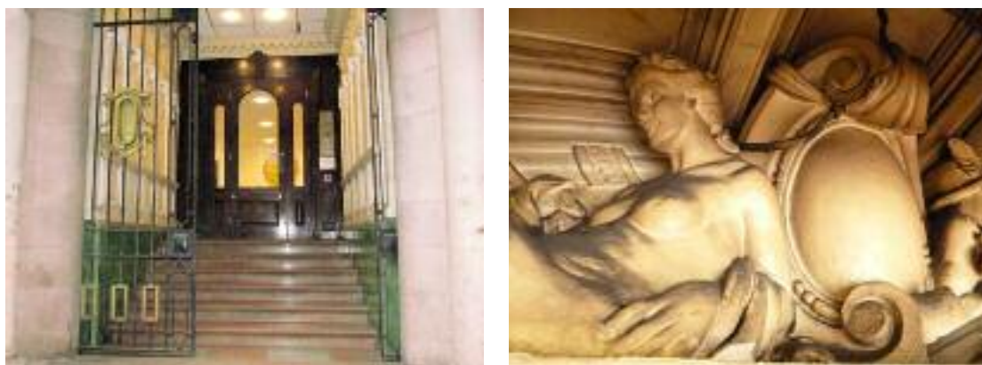
Figure 15: One of the two entrances (L) and rich plaster sculptural decoration above suspended ceilings (R)
