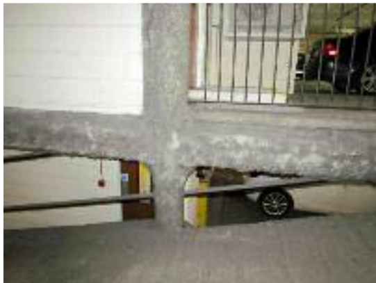
Figure 20: Modern fire-proof render on steel structure in Basement (L) and detail of riveted beam exposed below roadway (R)
