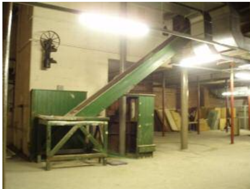
Figure 21: chute and lifting gear in Bridgewater House basement
