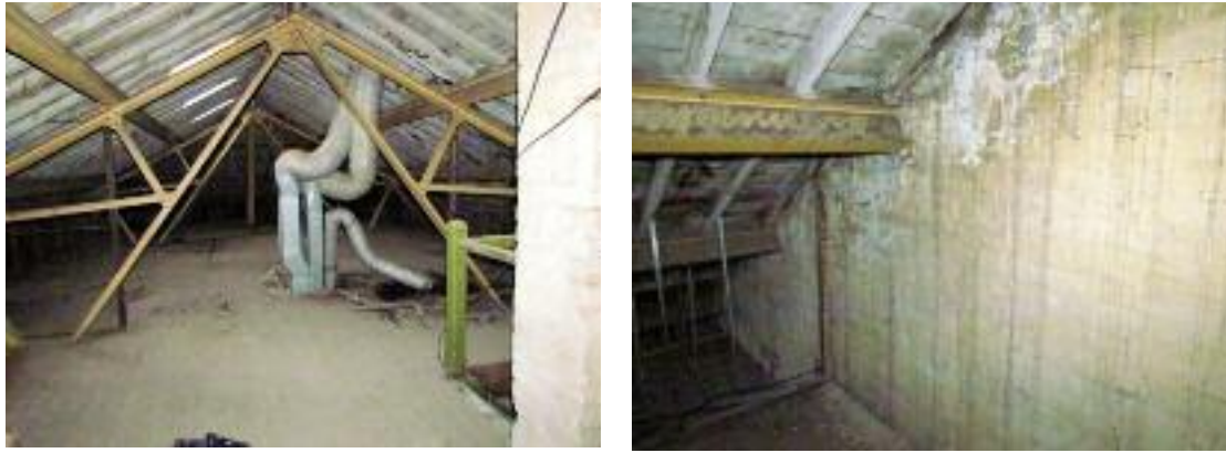
Figure 22: Steel roof trusses (L) and steel purlins (R)
