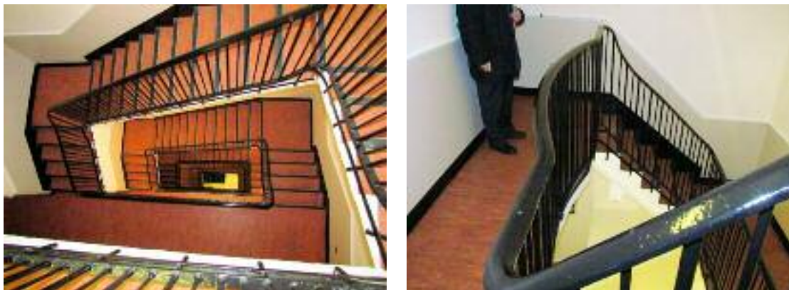
Figure 17: Vertical view of stairwell (L) and curved landing balustrade (R)
