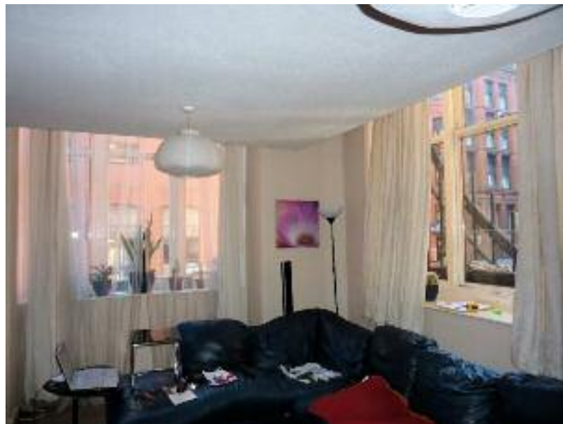
Figure 23: Suspended ceiling in a typical flat (photo courtesy of Warburton Associates)
