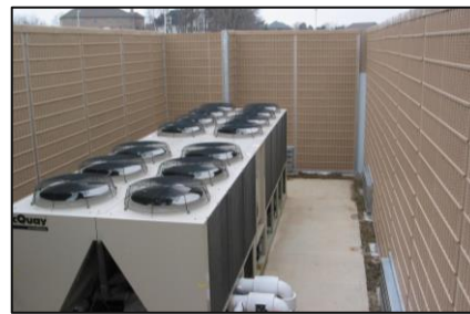
Figure 6—4 Acoustic barrier
