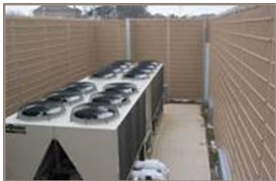
Figure 6—6 Noise barrier with acoustic lining
