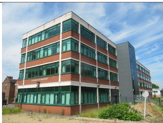
South-west and south-east elevations
