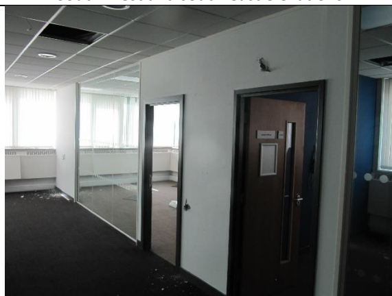
Internal former office space
