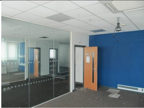
Internal former office space
