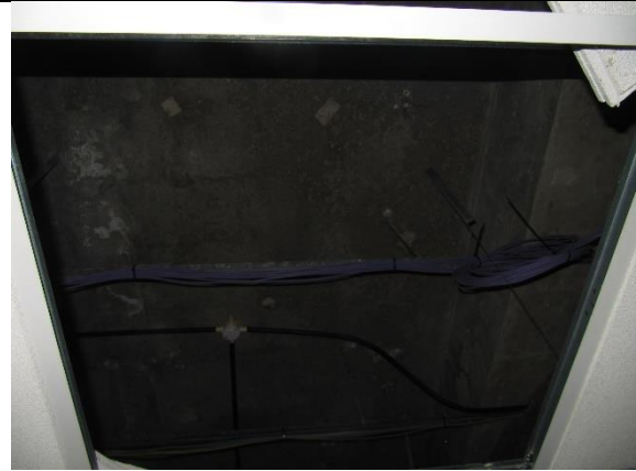
Suspended ceiling and space above
